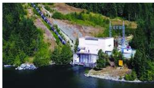
Photograph 2. Ash River Powerhouse. The penstock is visible behind the powerhouse.
