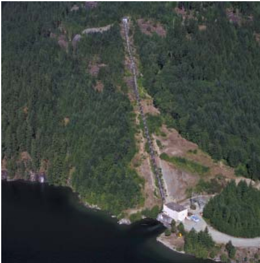
Photo 2-3: Ash River Powerhouse on Great Central Lake, 1999
