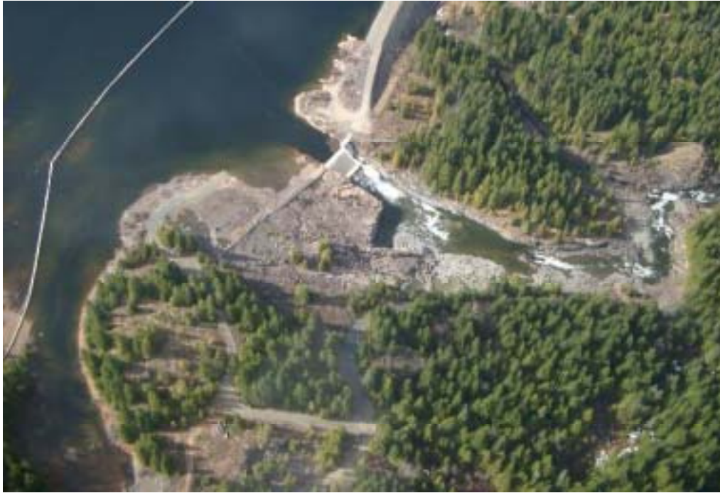
Photo 2-2: Elsie Lake Reservoir Overflow Dam with Overflow Spillway and Sluice Gate, 2002
