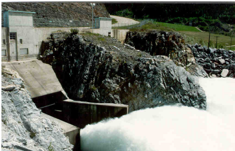
Photo 2-2: Duncan Dam Low-Level Outlets
