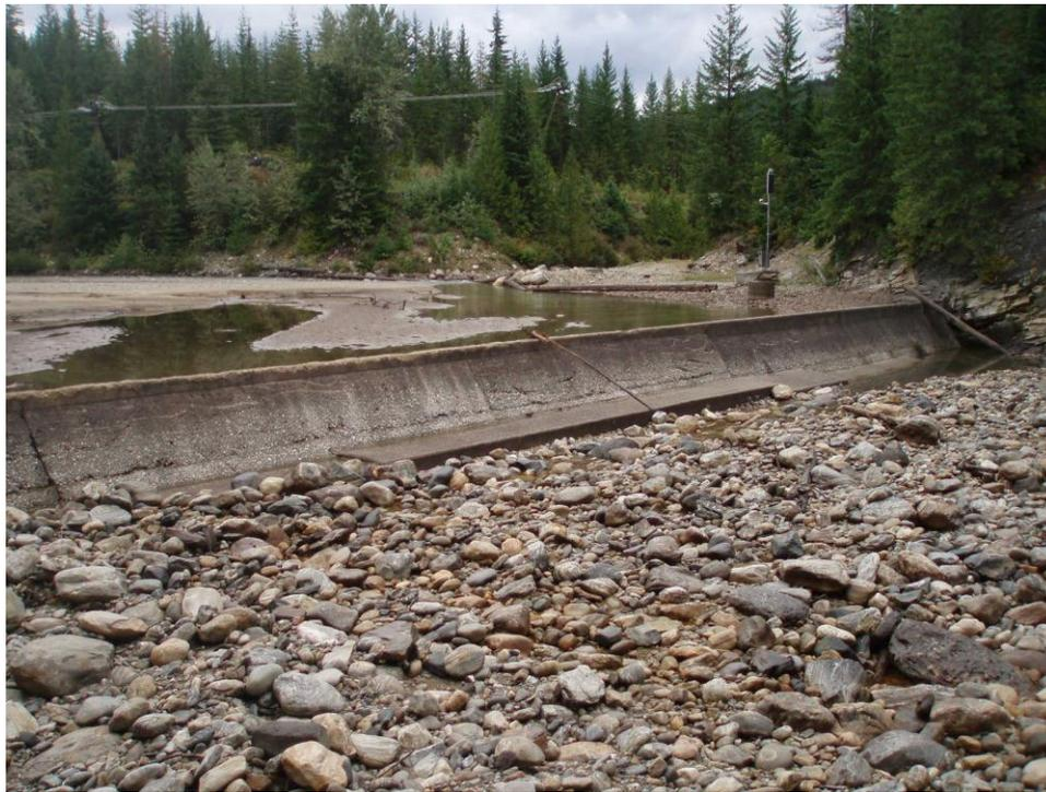
**Photo 3.** Dry conditions at the diversion dam. View from Lower Cranberry Creek downstream of the diversion dam facing upstream. Upper Cranberry Creek is located at the toe of the treeline and flows towards photo right into the Walter Hardman headpond. The minimum flow facility consists of two drywell intakes (perforated concrete cylinders) that are located on the right bank upstream from the diversion dam.
