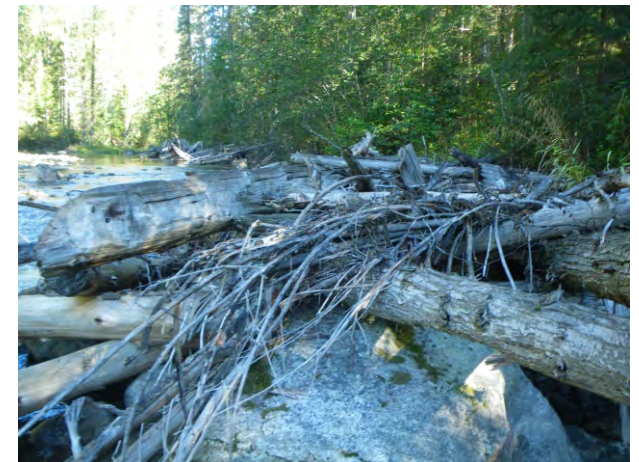
Photo C: Looking upstream at Structure 2 showing large recruited log and smaller debris. High water was close to top of structure.
