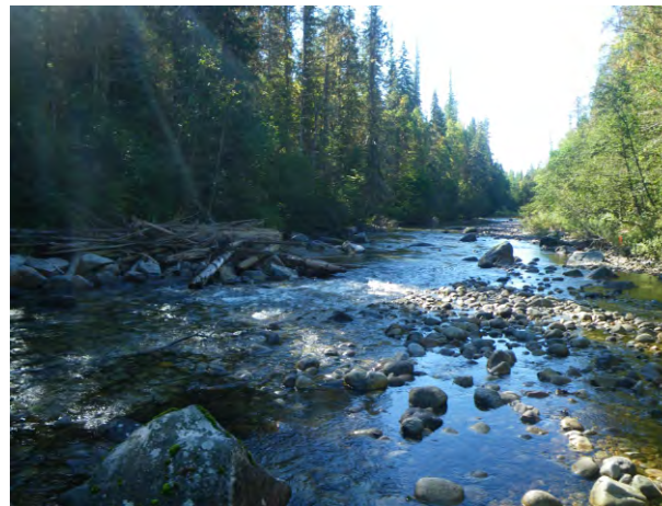
Photo B: Looking downstream at Structure 2. Note narrowed channel and increased velocity/scour off structure tip.
