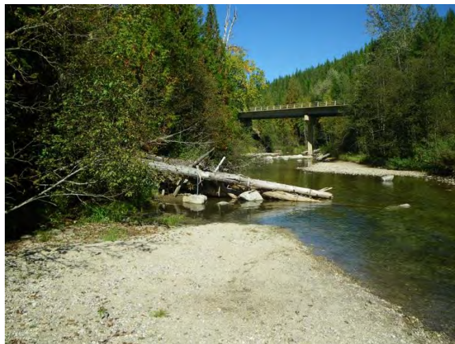
Photo C – Sand and gravel bar depositing downstream of Site 26. Structures and lateral bars are forcing stream meanders within the oversized channel.
