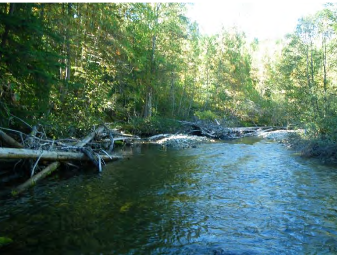
Photo K – Looking upstream from the bedrock constriction at Site 30. The near log jam is constructed and the far log jam is natural.
