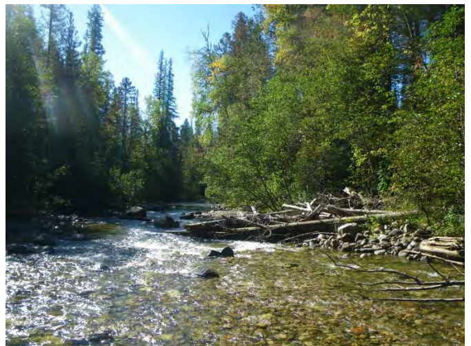
Photo D – Channel narrowed by a debris jam structure (Site 6) working in conjunction with large boulders to increase channel complexity.
