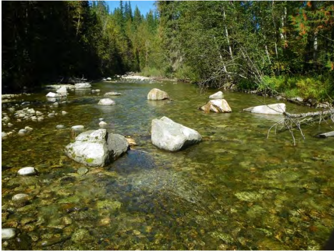
Photo G – Instream boulder placements downstream of Site 16. Minimal cover, scour and deposition of fines.
