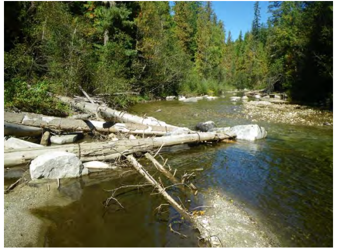
Photo B – Triangular rock and debris jam (Site 22) causing substrate sorting and deposition of sands, gravels and fines. Debris jams were set to force channel
