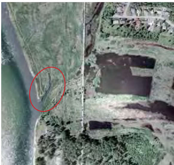
Erosion Channel at Airport Slough Outflow
