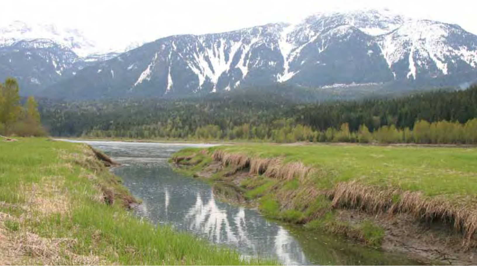
Airport Outflow Erosion Channel
