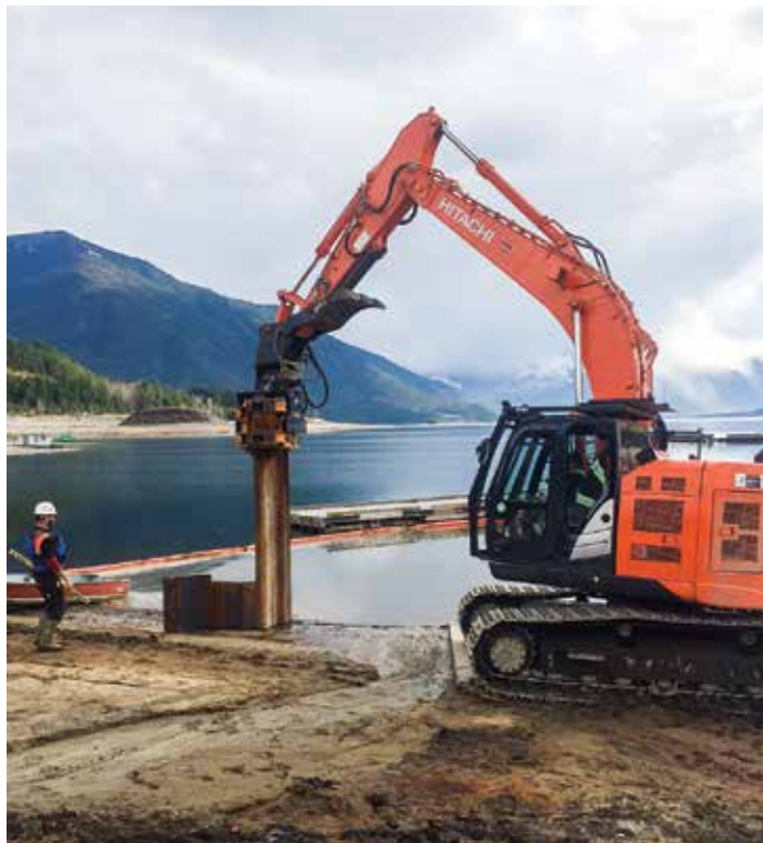
Building coffer dam at Nakusp to allow boat ramp panel installation.
