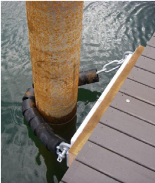
Boat ramp floating walkway.
