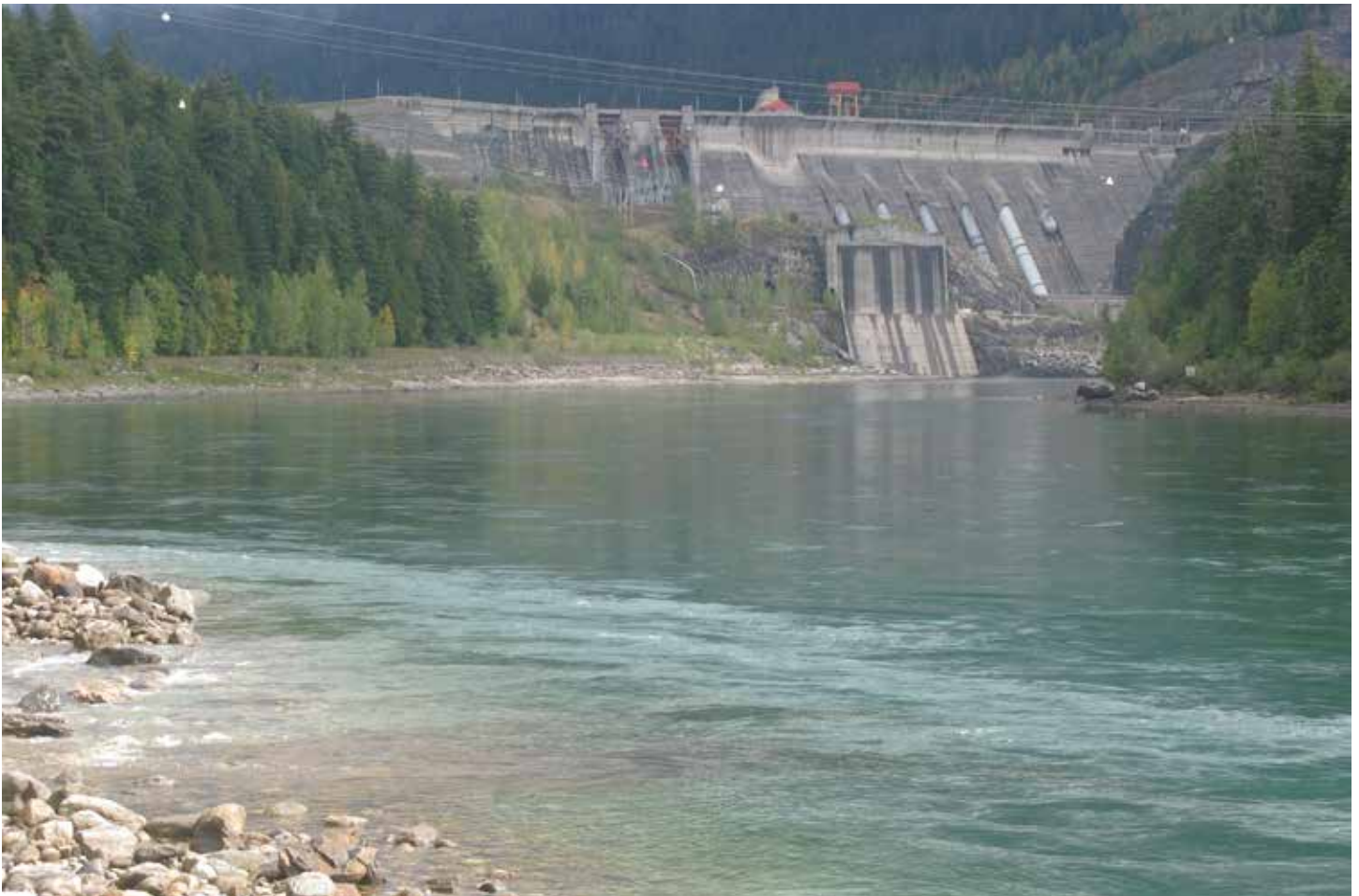
Revelstoke Dam & Generating Station.
