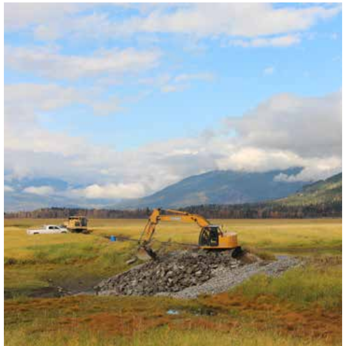
Heavy equipment places rock rip-rap to reinforce the collapsed culvert.
