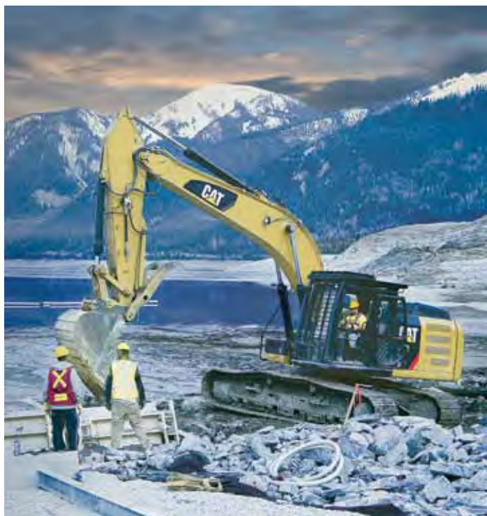
Bush Harbour boat ramp construction, April 2013
