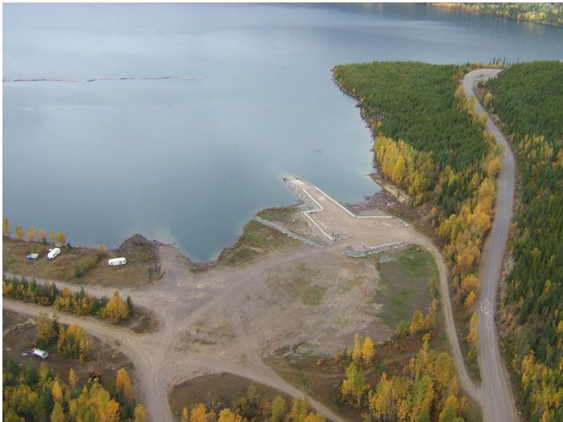
Figure 1: Bush Harbour boat launch; October, 32011. Reservoir elevation: 754.05m Lat: 51° 45' 23.043" Long: -117° 34' 26.8242"
