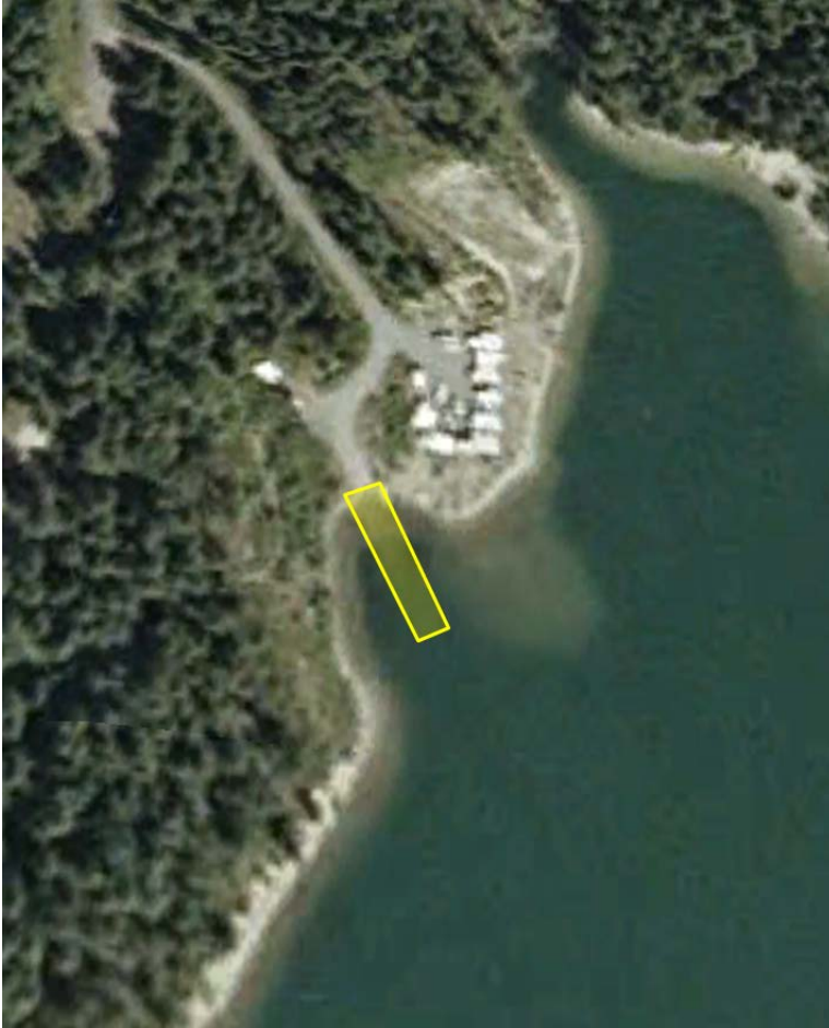
Figure 3: Downie Creek boat launch. Yellow highlights represent BC Hydro's area of responsibility for facility maintenance.
