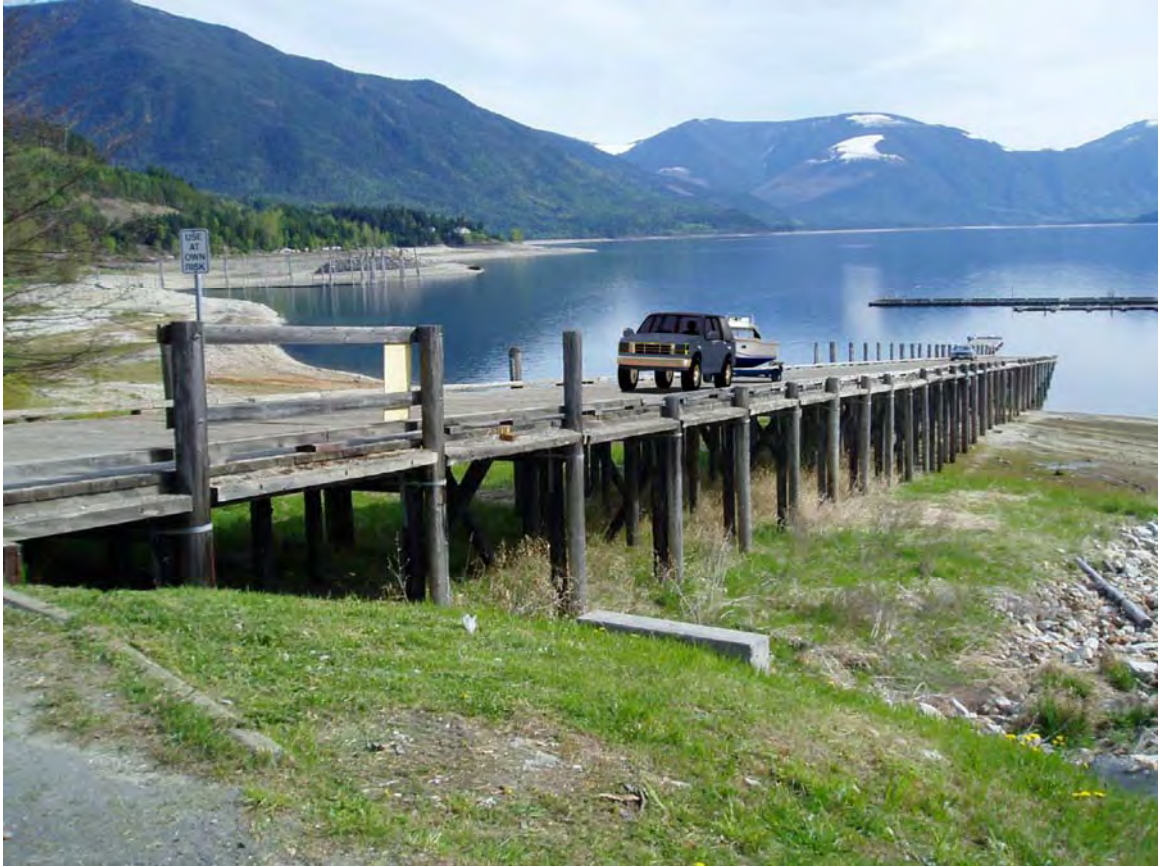
Figure 4.1 – Existing Timber Trestle Boat Launch Ramp
