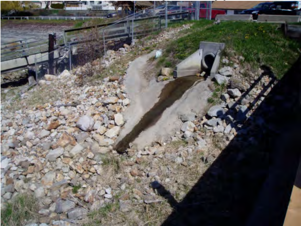
Plate 13. View of the storm drain outlet at existing Nakusp boat ramp.
