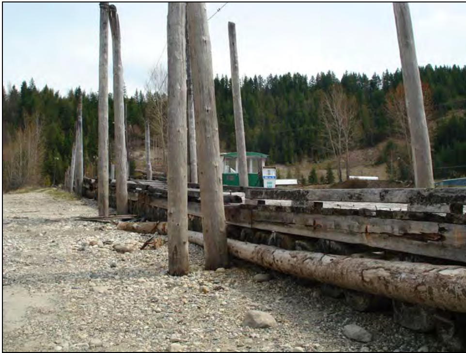
Photograph No. 38: Close-up view of derelict timber walkway floats
