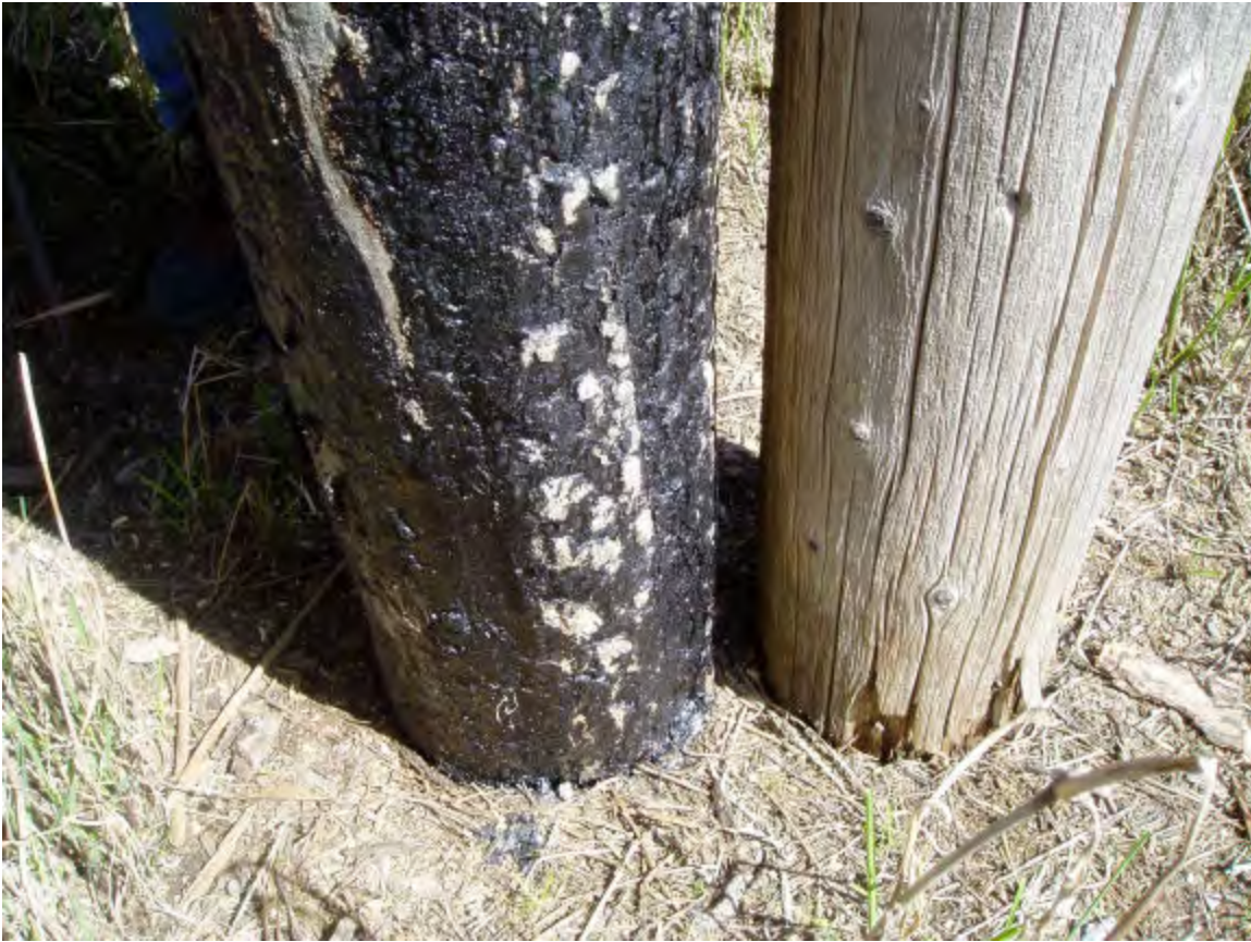
Plate 12. Treated timber piles used on inside of bridge but outside edge piles are untreated.
