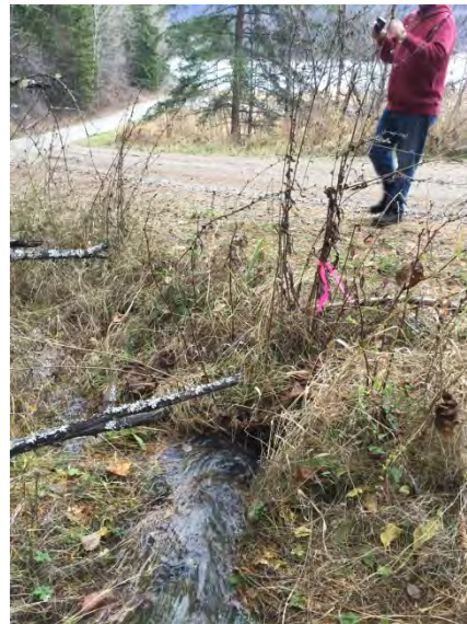
Photo 14: Culvert 4 on Lower Inonoaklin Road (channelized flow upstream)
