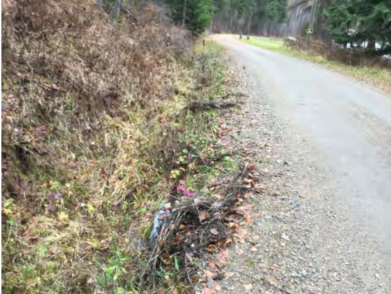
Photo 1: Culvert 3 on Lower Inonoaklin Road (south of residence)
