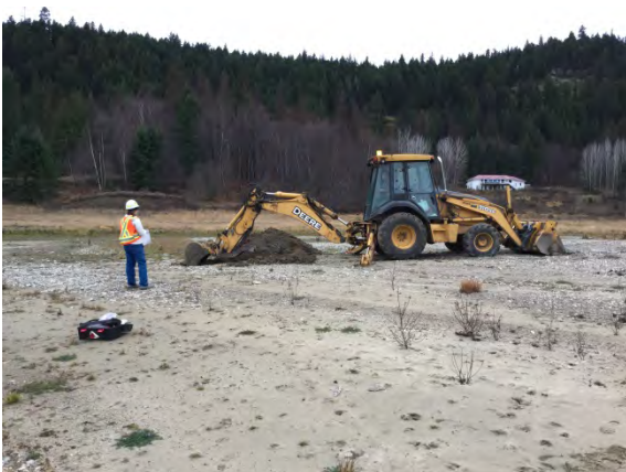
Photo 9: Test Pit 5 Near Proposed North End of South Berm
