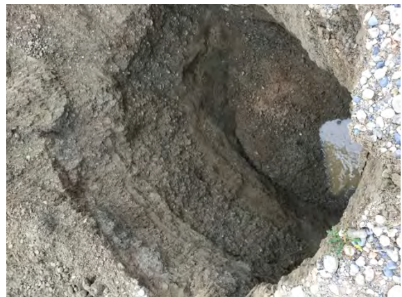
Photo 10: Test Pit 5 Near North End of South Berm
