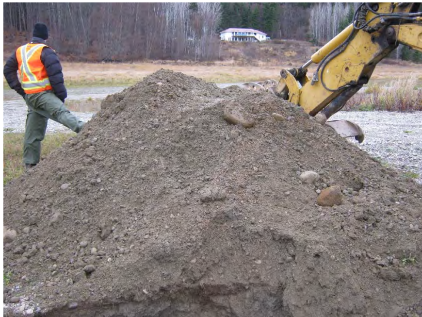
PHOTO 8: TP16-5 excavated material.
