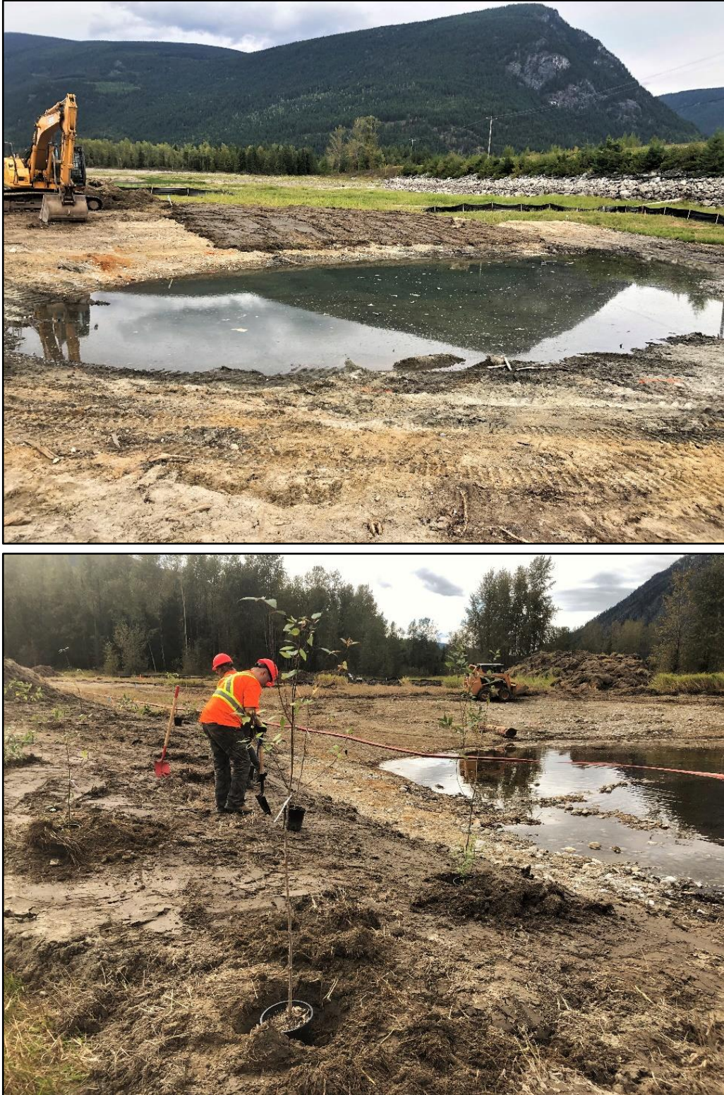
Figure 3-6. Top: application of topsoil at pond B1. Topsoil is comprised of overturned reed canarygrass sod. Bottom: Hand-digging planting holes in sod substrate for rooted cottonwood stock. Photos: M. Miller.
