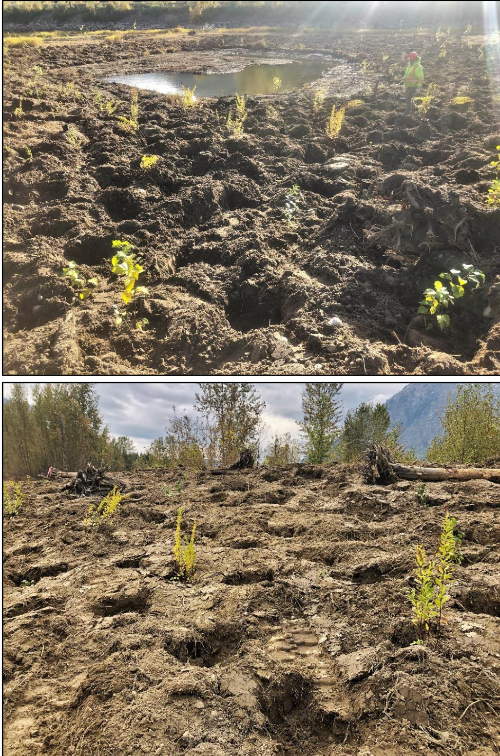
Figure 3-7. Examples of heterogeneous surface topography resulting from hole creation by mini excavator. Top: Partially planted bank of pond A2. Bottom: partially planted slope of mound C2. Photos: M. Miller.
