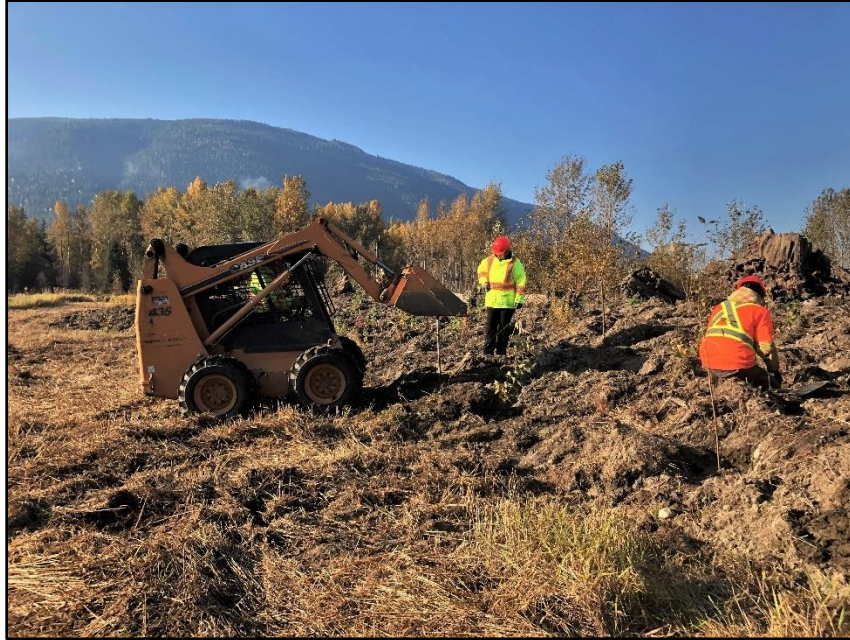
Figure 3-5. Creation of planting holes for live staking using a skid steer and iron bar. Photo: Mike Miller
