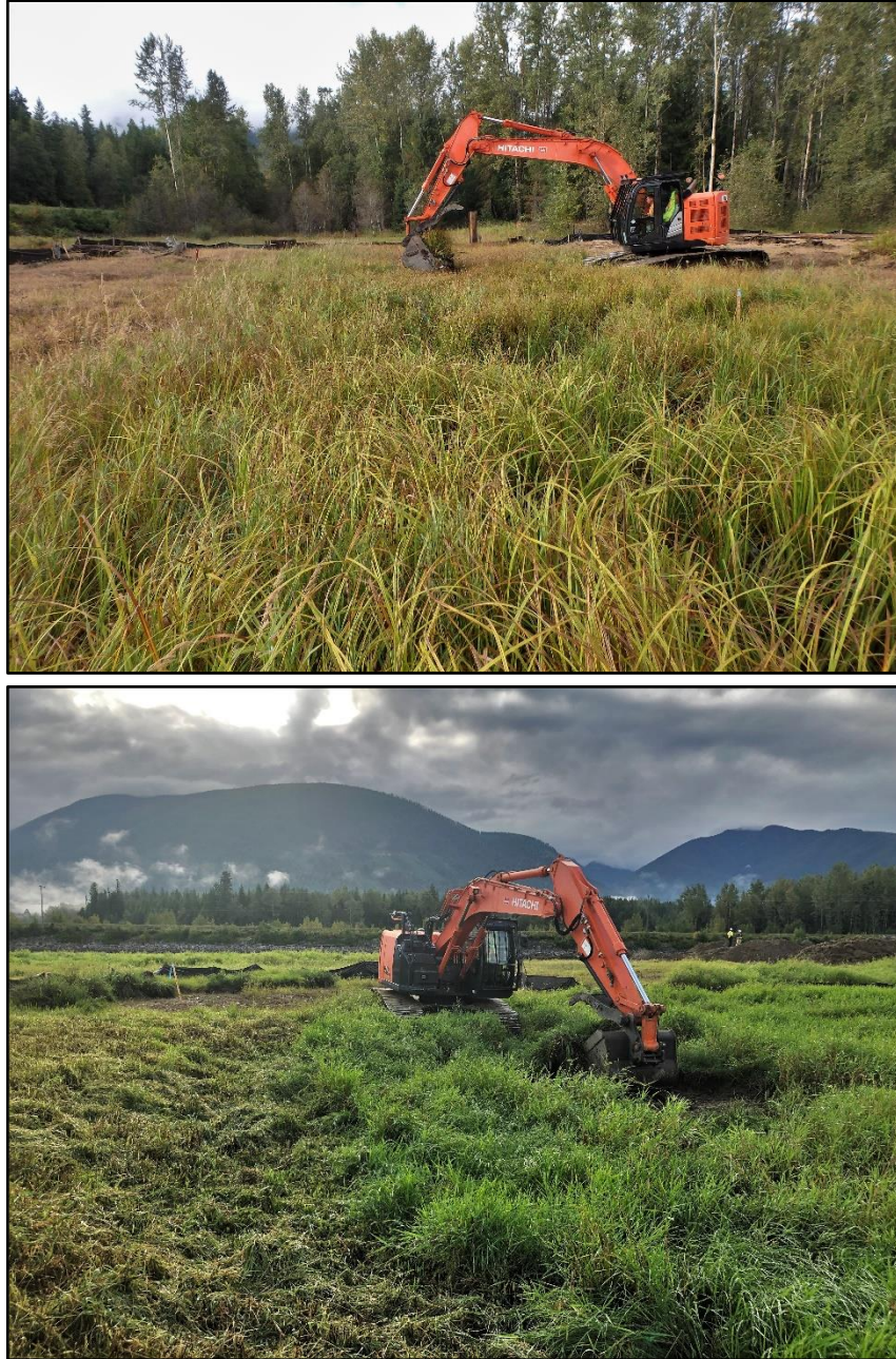
Figure 3-2. Native plant salvage with excavator. Top: stripping of wetland vegetation from the footprint of pond A1. Bottom: stripping Kellogg's and Columbia sedge sod from the footprint of pond B1. Photos: M. Miller.
