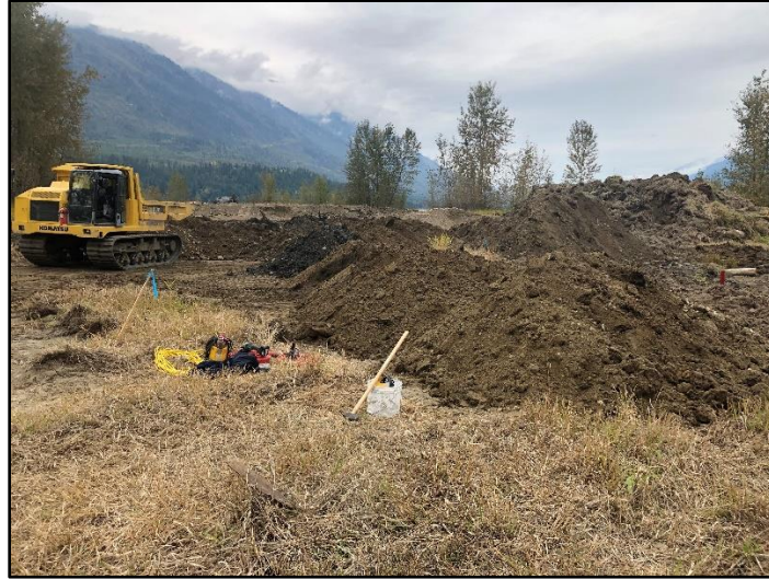
Figure 3-8. Stockpiled subsoil from pond A1 used to backfill planting holes. Photo: M. Miller.
