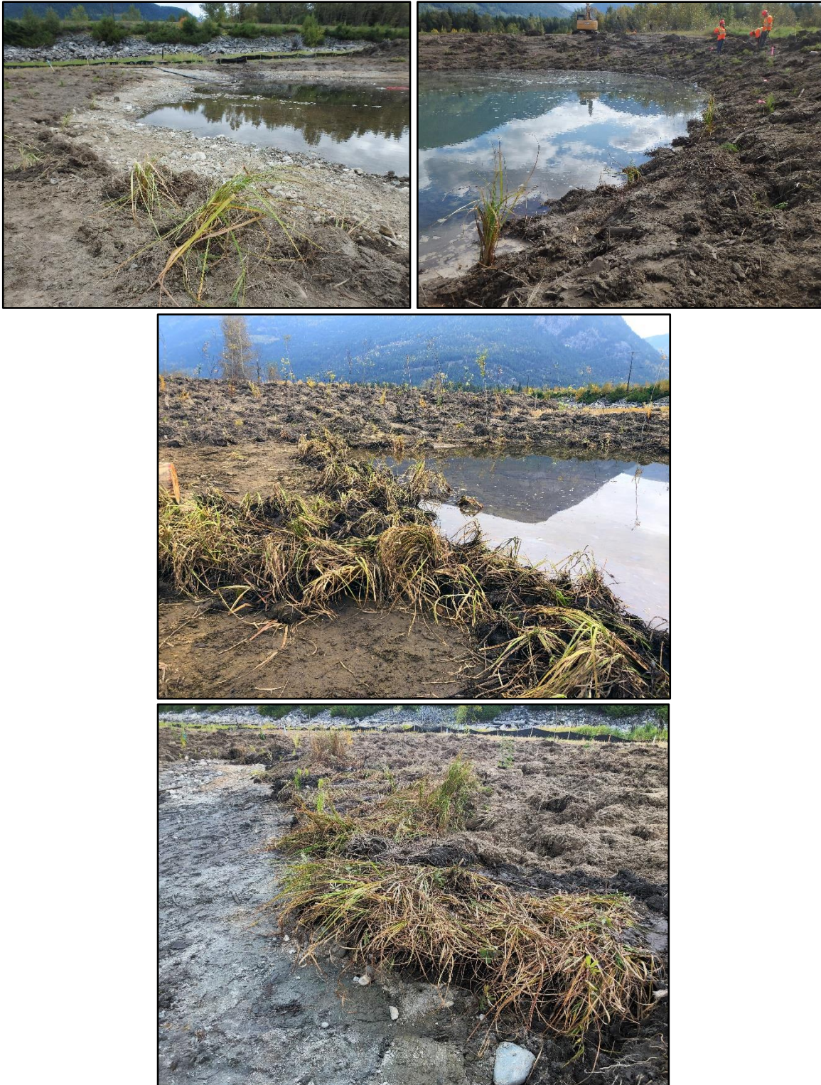
Figure 3-9. Top: trial transplants of salvaged beaked sedge plugs at the projected water lines of ponds A4 (left) and B1 (right) and in the projected littoral zone of pond A2 (middle). Bottom: machine-placed wetland salvage mix (beaked sedge/bluejoint reedgrass/small-fruited bulrush sod) at the projected waterline of pond A2. Photos: M. Miller.
