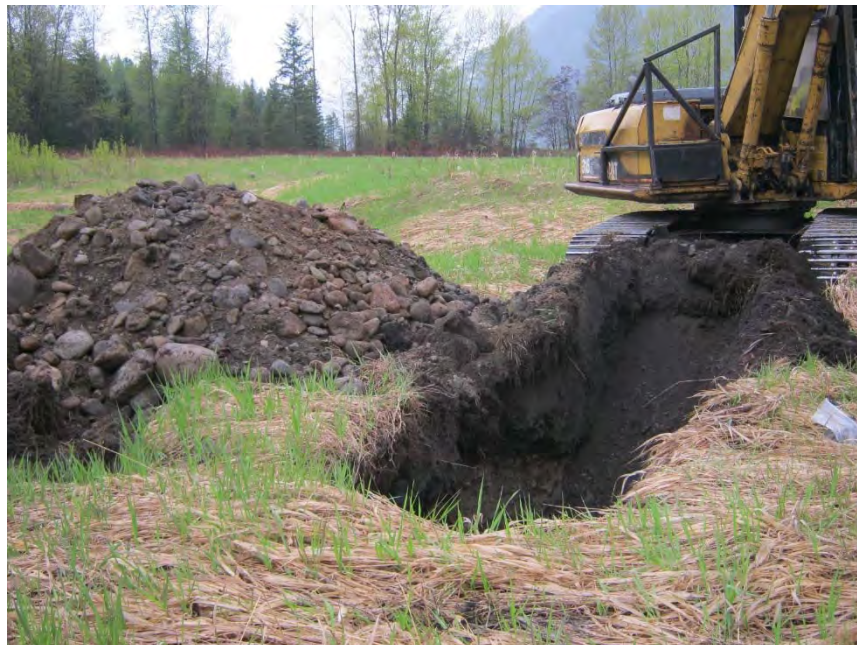
PHOTO 2: Excavation of TP17-2.
