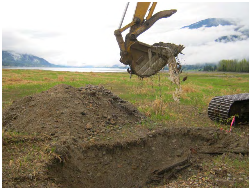
PHOTO 6: Excavation of TP17-6.
