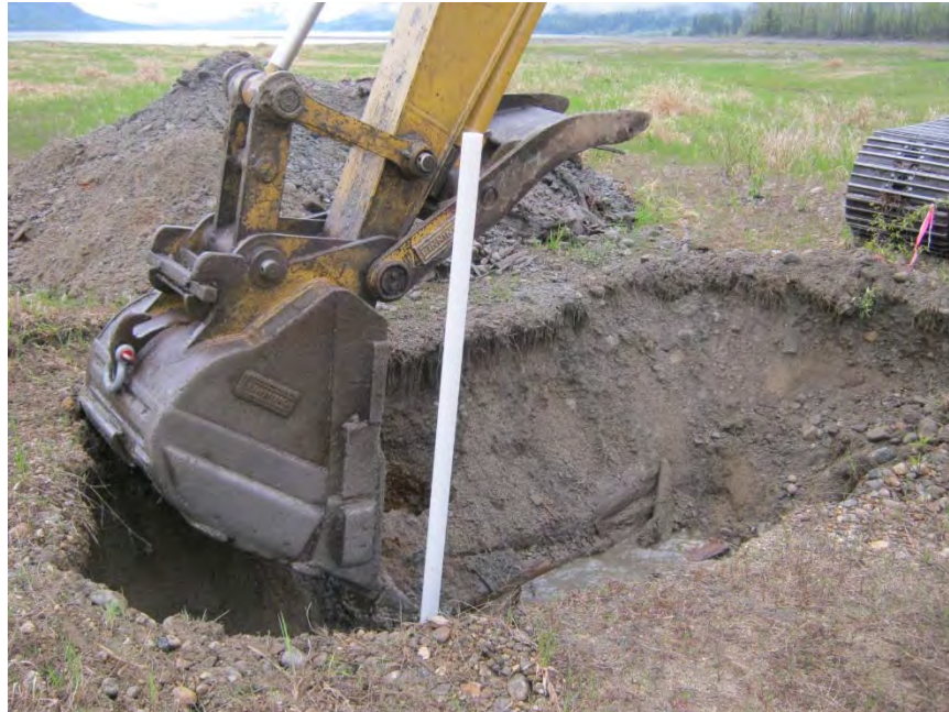
PHOTO 7: Piezometer installation at TP17-6.
