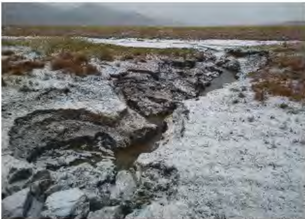
Photo 11: Looking north along eroded channel at Area B. Evidence of previous head-cutting in erodible floodplain silts.
