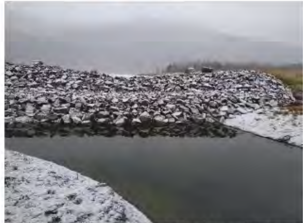
Photo 14: Looking east at Site 15a outlet from downstream side.
