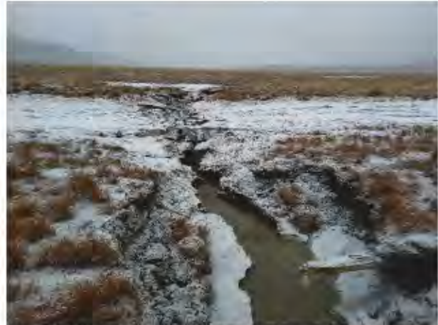
Photo 10: Looking north along area B. Riprap was placed in the eroded channel to partly re-establish the road.
