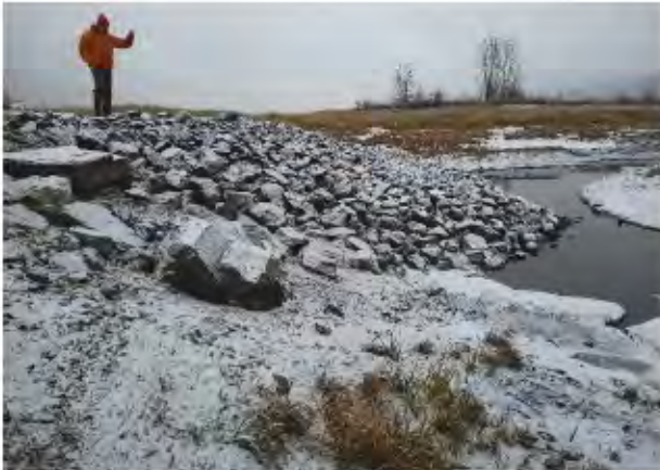
Photo 13: Looking south. Riprap facing on downstream side of Site 15a Dam.
