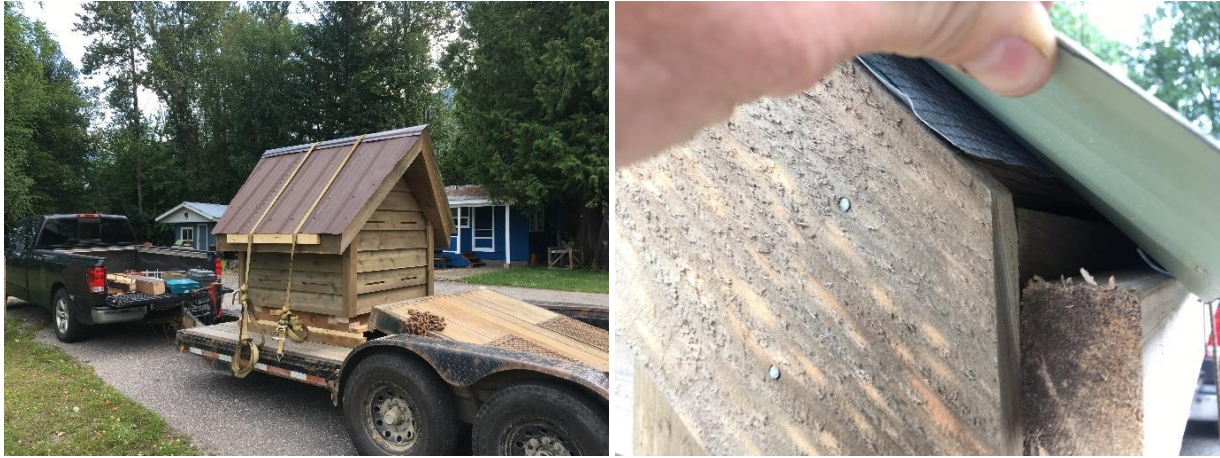
Figure 5. The modified mini-condo (left) was purposefully built with a number of gaps to provide multiple access points for bats while still being weatherproof, such as this side access port under a loose piece of tin roofing (right).
