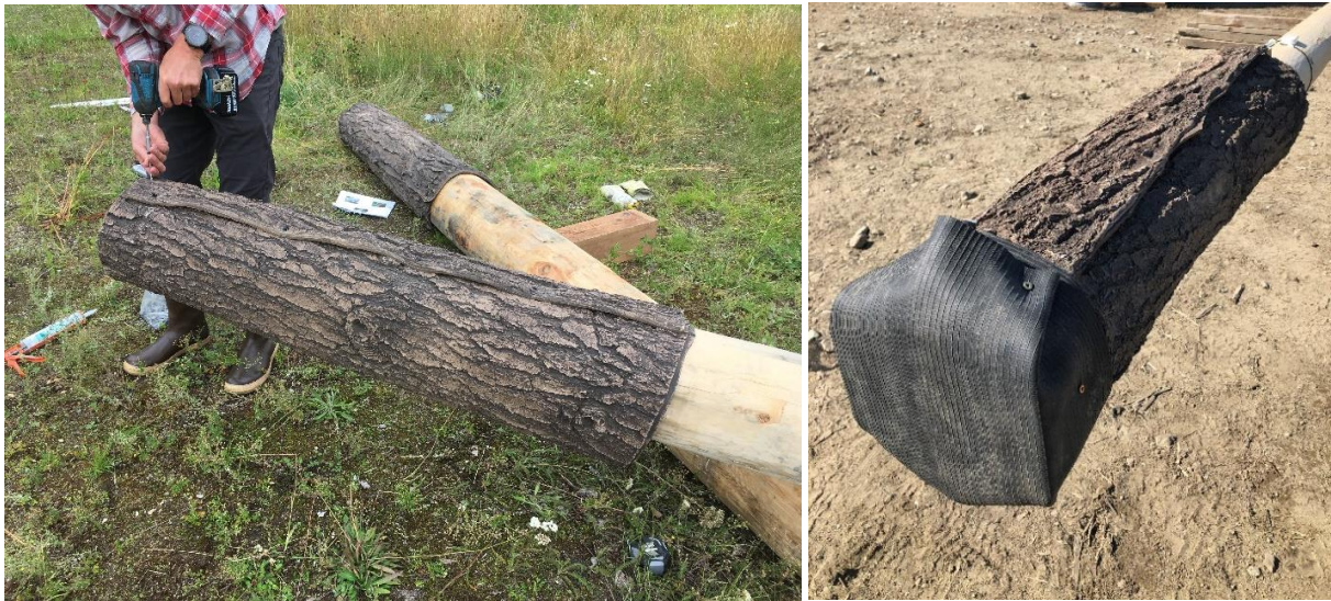
Figure 7. BrandenBark sheets were wrapped around pole tops as per the manufacturer's instructions. The top seam was caulked, and then the two Hay Field and Burton poles also had the surface covered with rubber or extra BrandenBark pieces for extra weatherproofing.
