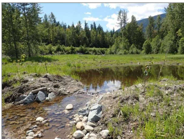
Photo 3. View of A1 outlet looking south, June 18, 2020.
