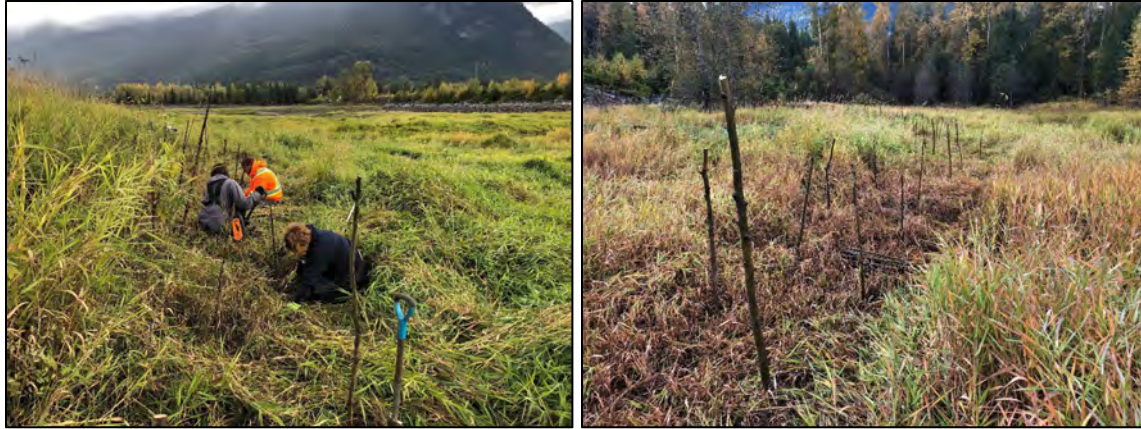
Figure 3-8. Live staking with black cottonwood. Left: Staking between mound C2 and pond A3. Right: installed stakes above pond A2. Photos: M. Miller.
