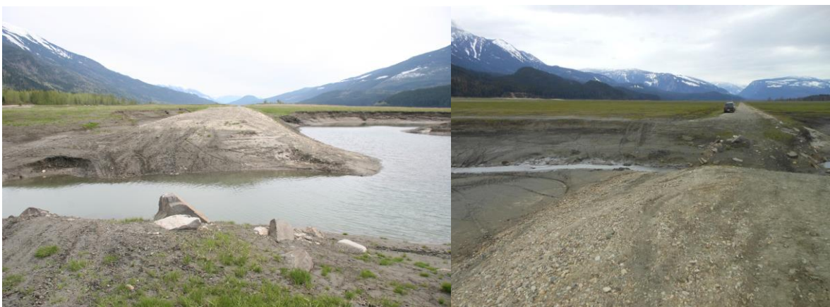
Figure 1: Site 14 gap in the rail bed looking North allowing water to pass into Cartier North in October 2013, (el 432.1 m) on the left and May, 2012 (el. 430.7 m) on the right
