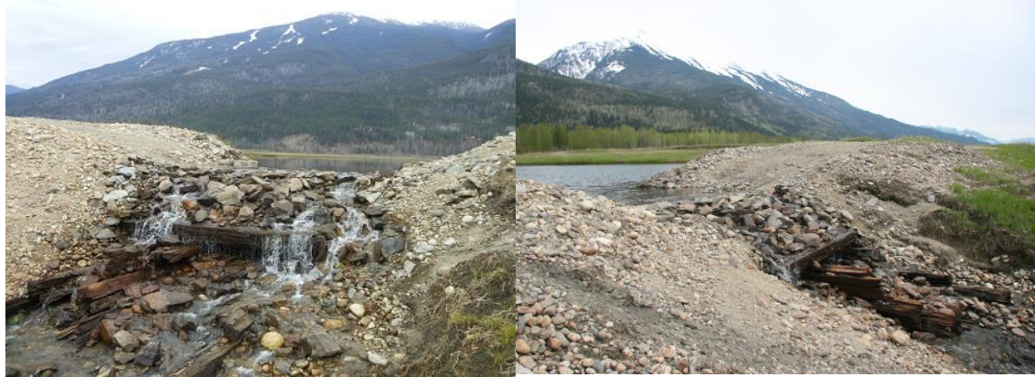
Figure 2: Site of the wood-box culvert at Site 15A, el. 429.9 m (May 7, 2015)
