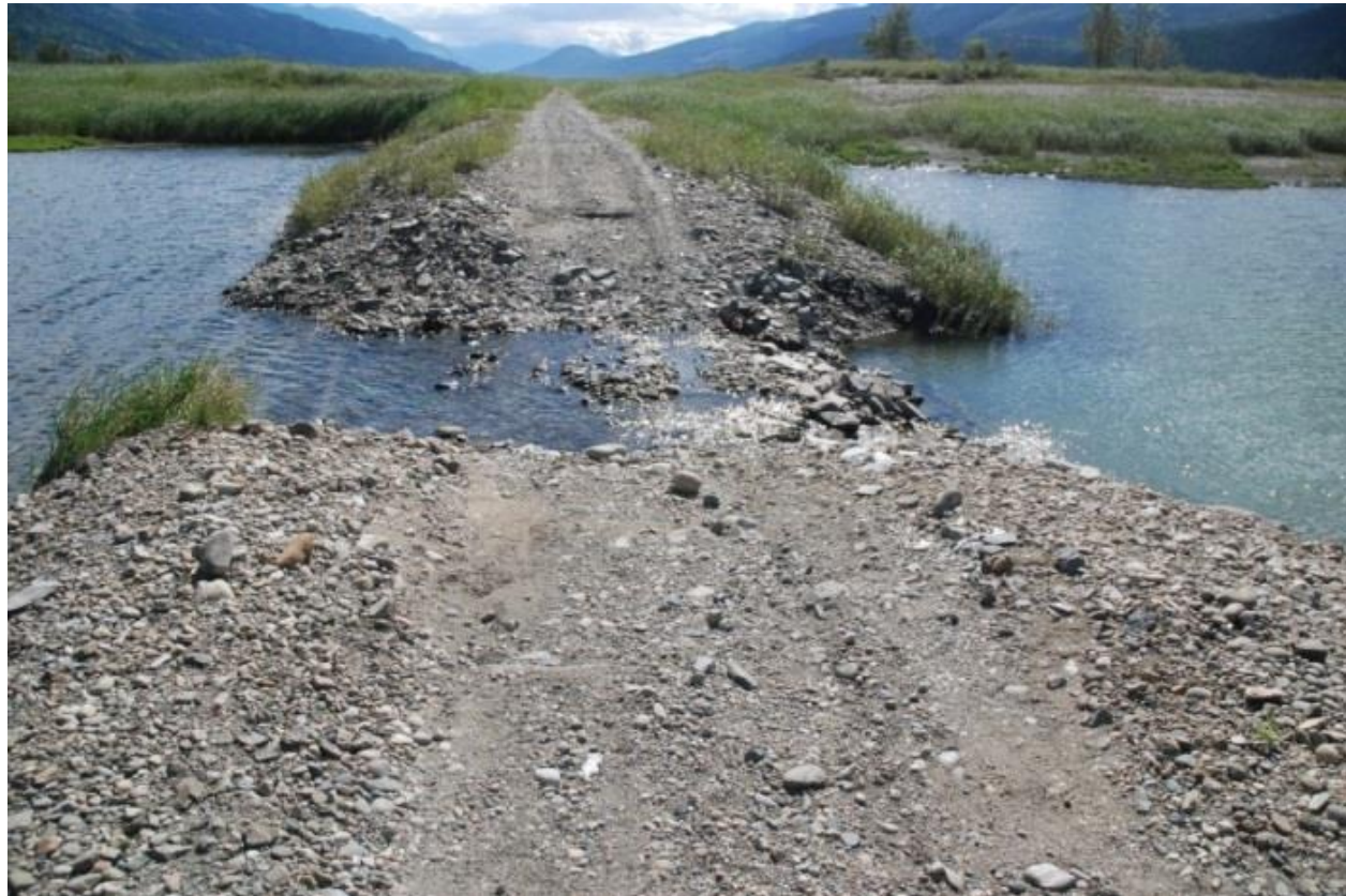
Photograph 3. Site 15A consists of collapsing wooden culvert that has created a gap in the old rail grade north of Site 14. This area would also be rebuilt with a raised invert.
