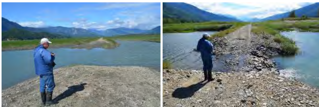
Figure 4-5. Current photos of Site 14 (left) and 15A (right), Cartier Marsh box culvert and swale outlet (September 8, 2014, reservoir elevation 433.62 m ASL)
