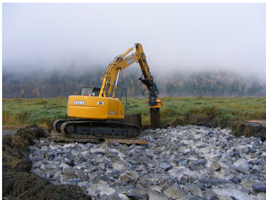
Photograph 13: Extracting sheet piles.
