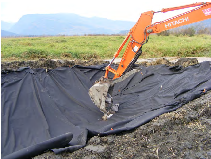
Photograph 5: Commencing placement of rip rap.
