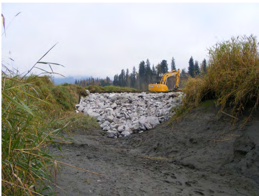
Photograph 16: Downstream end of rip rap.
