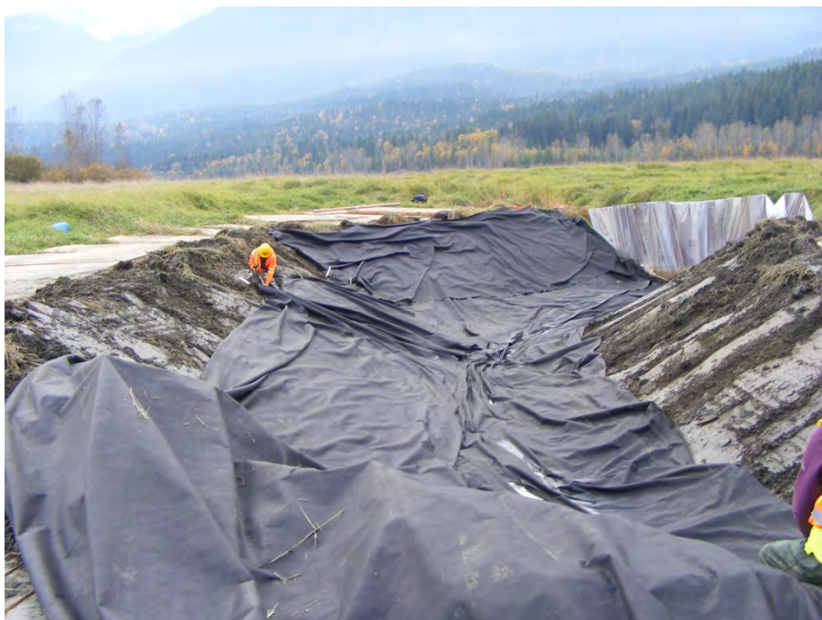
Photograph 3: Placing geotextile.
