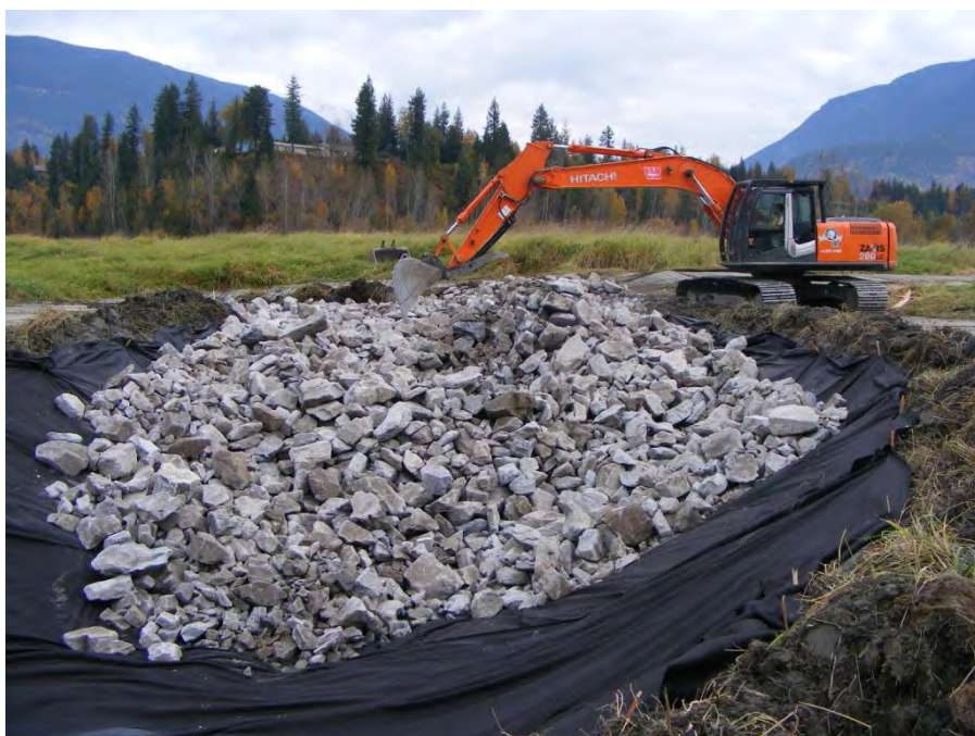
Photograph 8: Most rip rap replaced.
