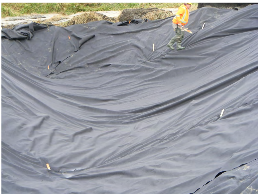
Photograph 4: Geotextile placement completed.
