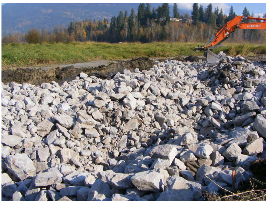
Photograph 11: Completion of trimming rip rap.
