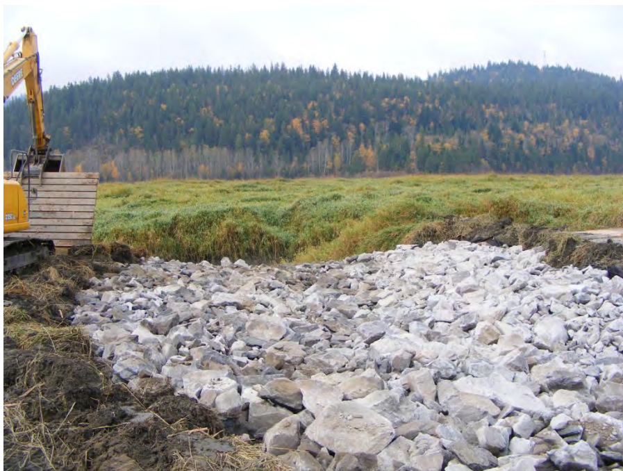
Photograph 15: Downstream end of surface rip rap with steel sheet piling removed and removing swamp mats.
