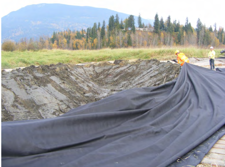
Photograph 2: Commencing placement of geotextile.
