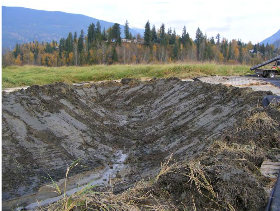
Photograph 1: Muck removed from the channel perimeter, grass stripped off and site prepared for geotextile.
