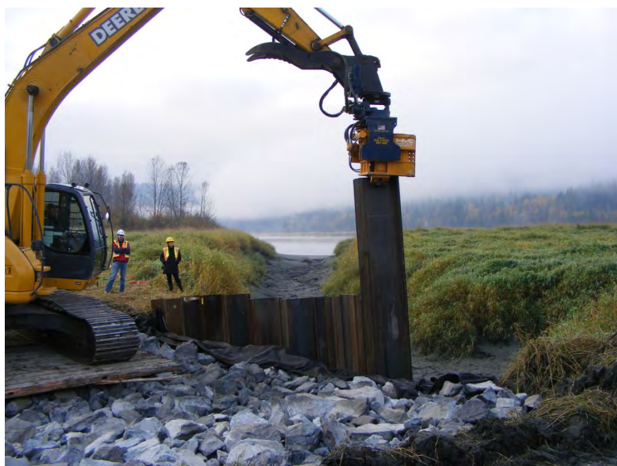
Photograph 14: Extracting sheet piles.
