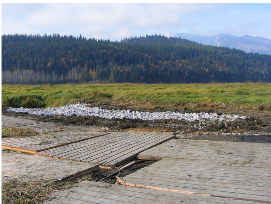
Photograph 17: Completed rip rap and some removed swamp mats.
