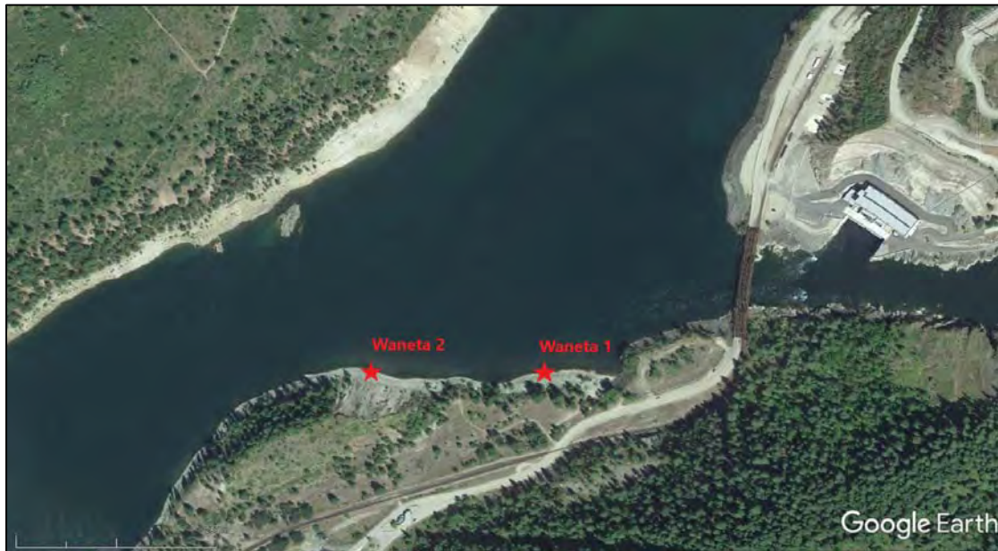
Figure 5 Waneta Site Locations
