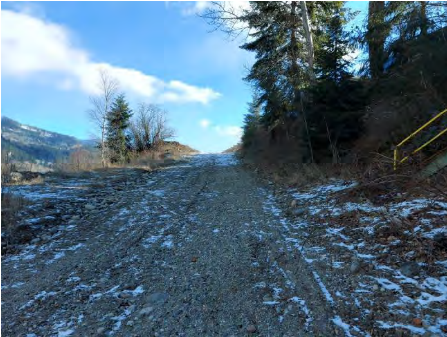
Photo 1: View east of the existing access road to the south bank laydown area and river access (12 February 2021).
