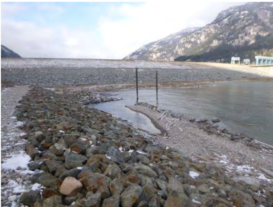
Photo 4: View west of the south bank laydown area and river access (12 February 2021).
