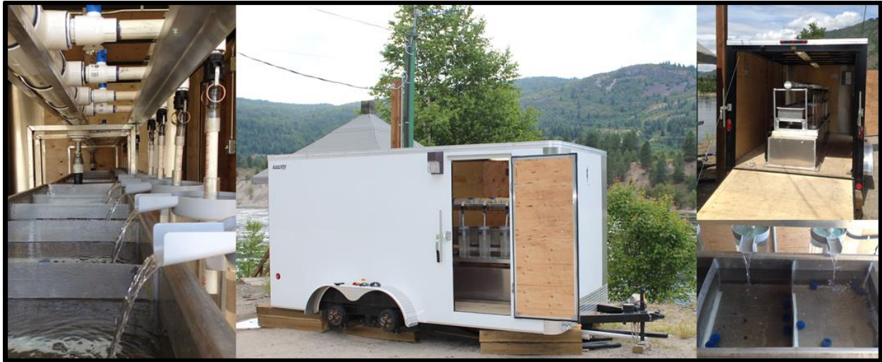
Figure 2. Streamside Incubation Facility (outfitted cargo trailer) used for rearing wild origin White Sturgeon progeny on the Columbia River.
