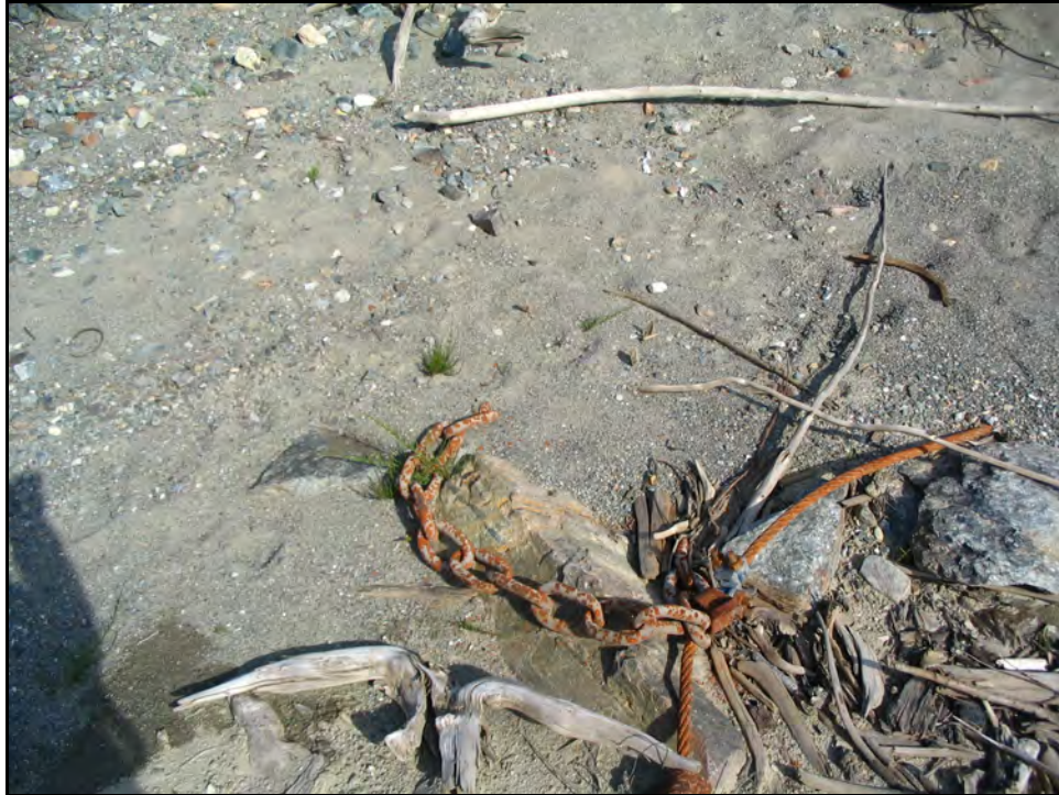
Photo No. 17: Taken on 2007-05-25 at Valemount Marina View of buried anchors, cables and chain anchors for floats.
