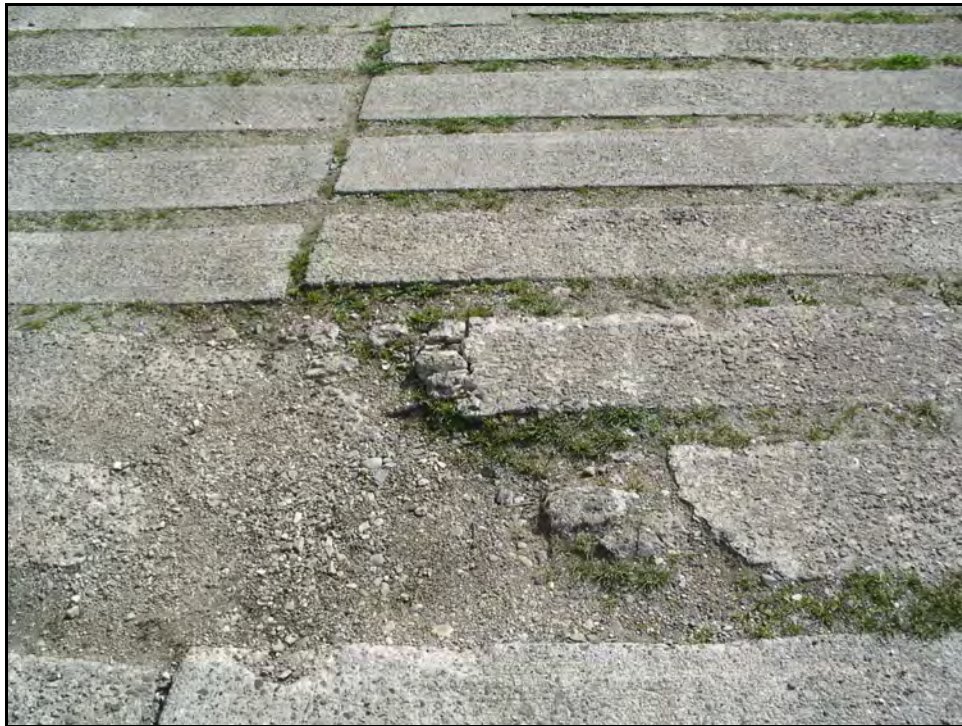
Photo No. 65: Taken on 2007-05-24 at Centennial Park Close-up view of damaged concrete planks in the boat launch ramp.
