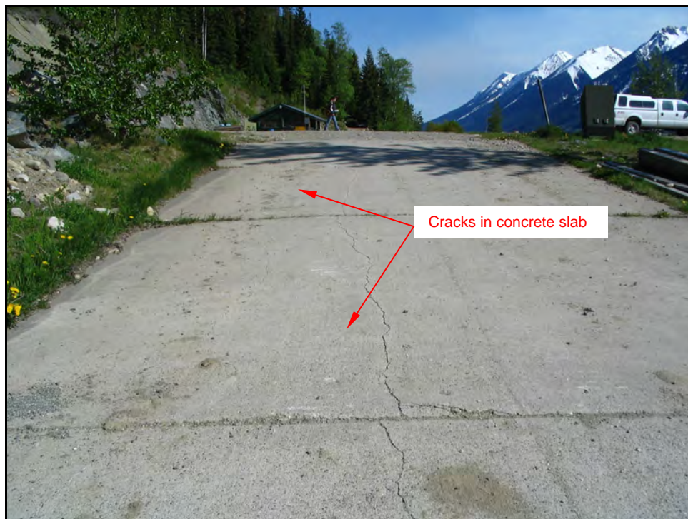
Photo No. 8: Taken on 2007-05-25 at Valemount Marina View of the boat launch ramp showing cracks along length of the concrete slabs.
