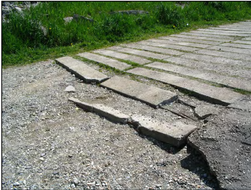
Photo No. 61: Taken on 2007-05-24 at Centennial Park Broken Concrete planks at the end of the boat launch ramp.
