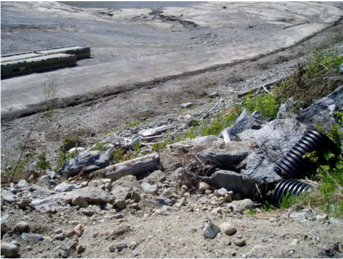
Plate 7. View of current ramp, ditchline and culvert conveying surface flow during spring freshet. Will need to incorporate these features into EMP.
