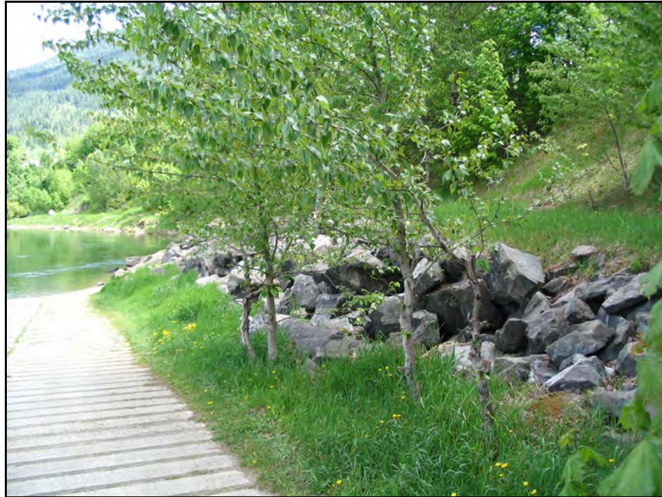
Photo No. 58: Taken on 2007-05-24 at Centennial Park View of the shore protection work along the side of the boat launch ramp.
