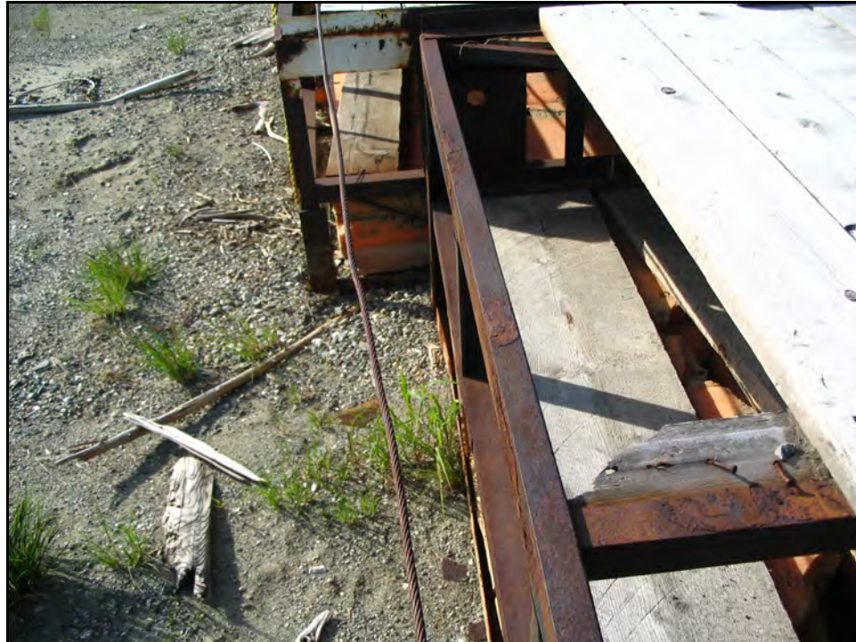
Photo No. 16: Taken on 2007-05-25 at Valemount Marina Close-up view of steel frame members for floats. Note rust build-up on uncoated steel frame members.
