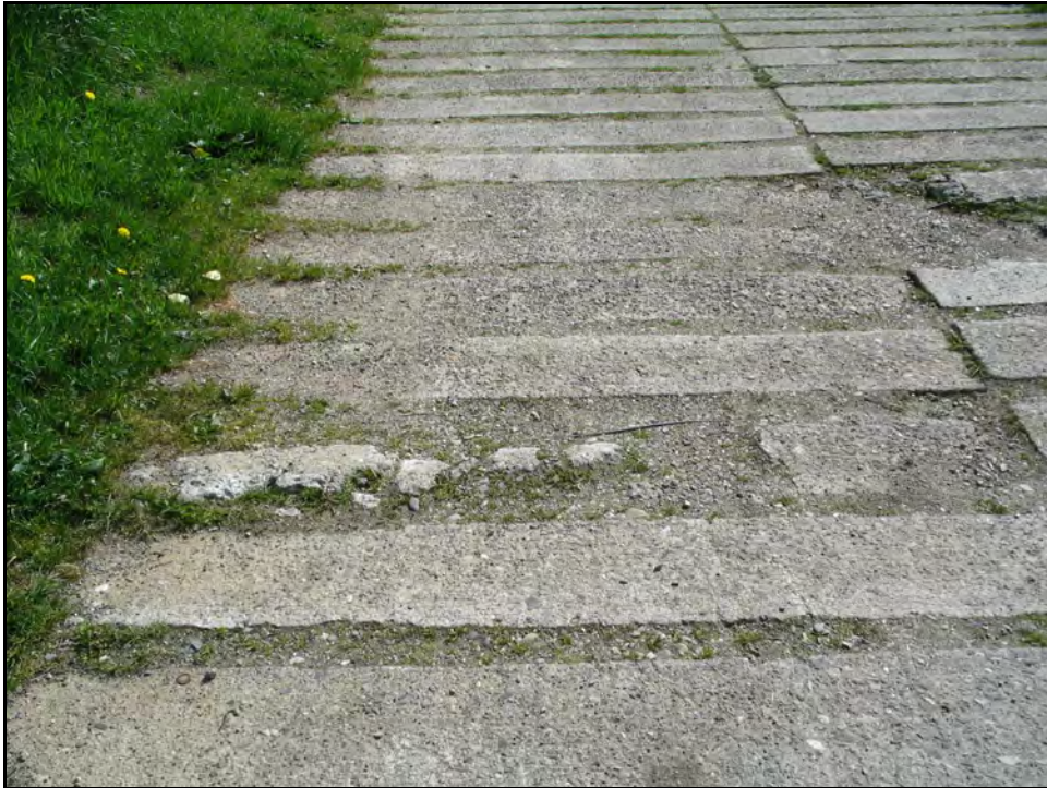
Photo No. 64: Taken on 2007-05-24 at Centennial Park View of the damaged concrete planks at section on the ramp.
