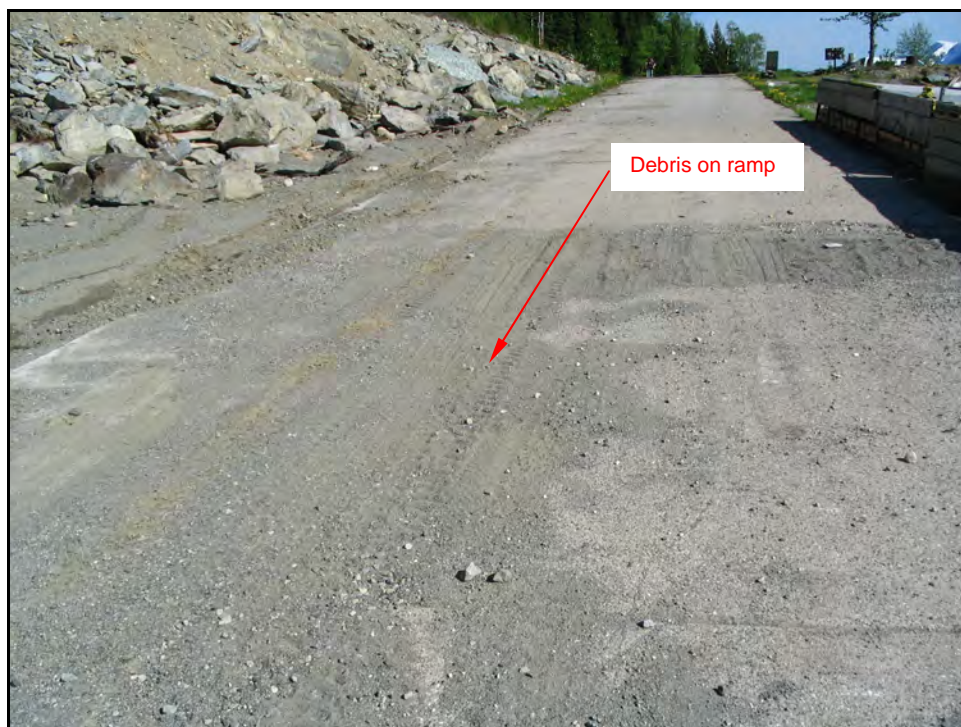
Photo No. 10: Taken on 2007-05-25 at Valemount Marina Boat launch ramp showing debris on the ramp from adjacent sloped area.
