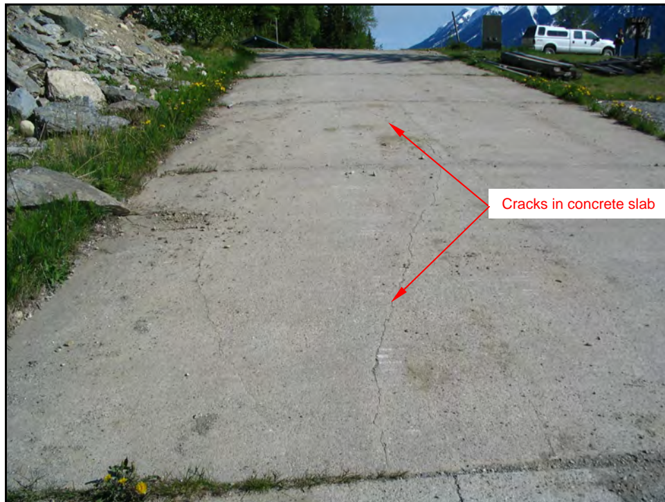
Photo No. 9: Taken on 2007-05-25 at Valemount Marina More cracks further along the ramp.
