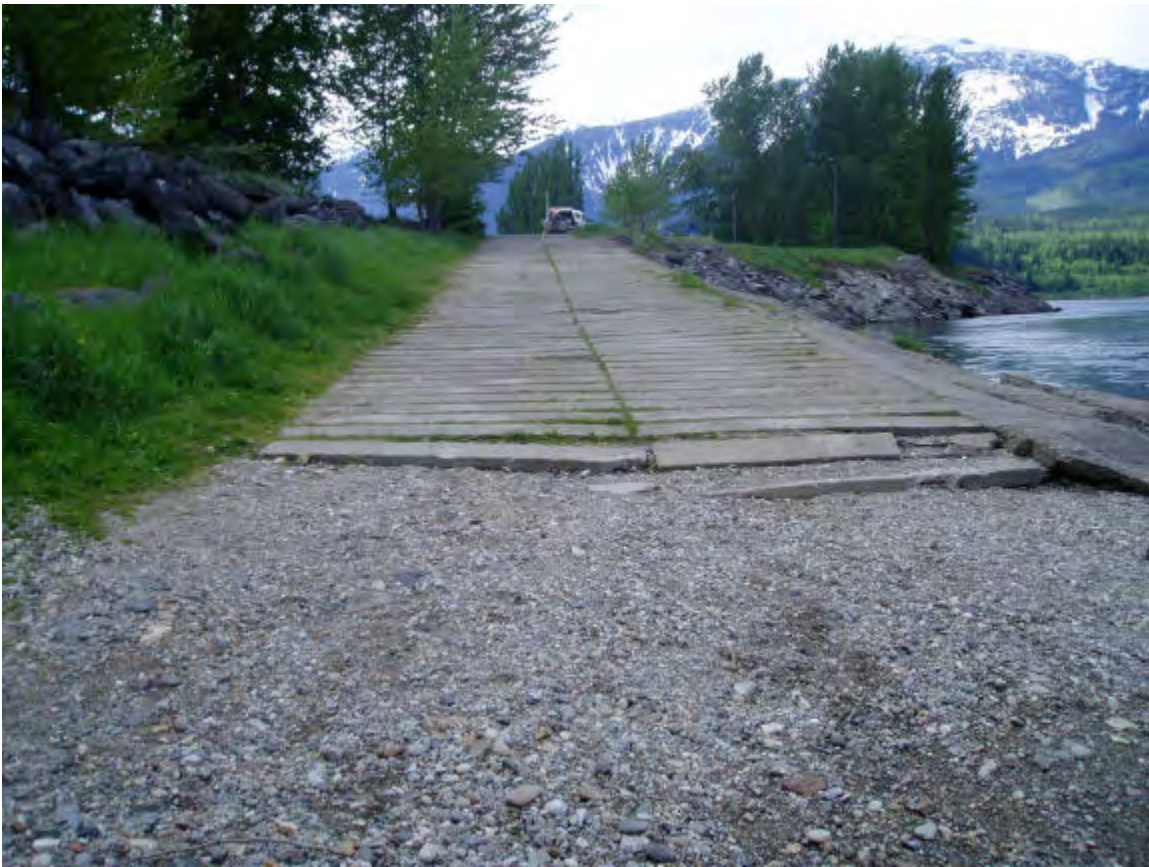
Plate 37. Looking southwest at current ramp conditions at Centennial Park. Note riprap bank protection downstream of ramp.
