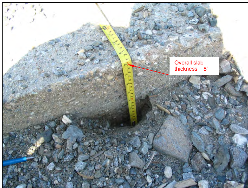
Photo No. 12: Taken on 2007-05-25 at Valemount Marina Close-up view showing the 8" thickness of the existing concrete slab.
