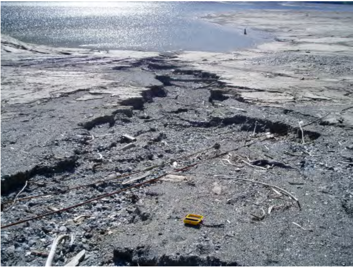
Plate 11. Looking east at extensive erosion caused by ditchline flows jumping the ramp.
