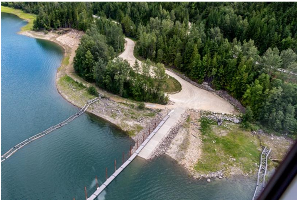
Figure 1: Aerial view of Burton South boat launch, 49°57'54.85"N 117°55'0.69"W, June 17, 2015; Reservoir elevation: 435.3 m (1428.1 ft.)
