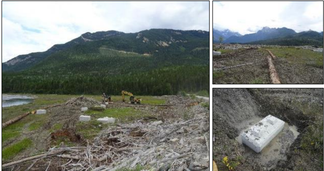
Figure 3-1: Installation of Log boom at Bush Causeway North, June 2016. Left: placing logs and lock block; top right: lining up logs; bottom right: burying lock blocks.
