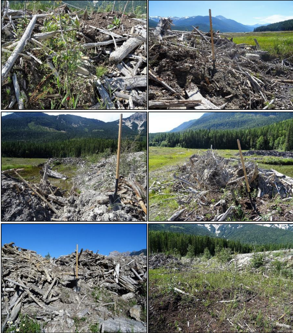
Figure 3-1. Constructed mounds, Bush Causeway (north site), illustrating current state of establishing planted and natural vegetation. Leaf-bearing live stakes are visible in the top left and bottom right panels. Photographed July 2018.
