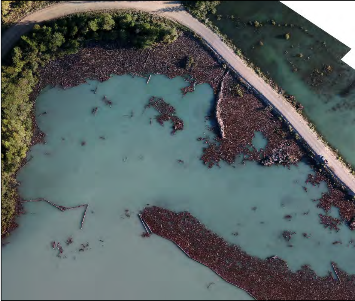
Figure 5. Aerial image of the log-boom breach at Bush Arm following a windstorm in August 2020. Image obtained by Murray Chapple, Sterling Lumber Co Ltd.
