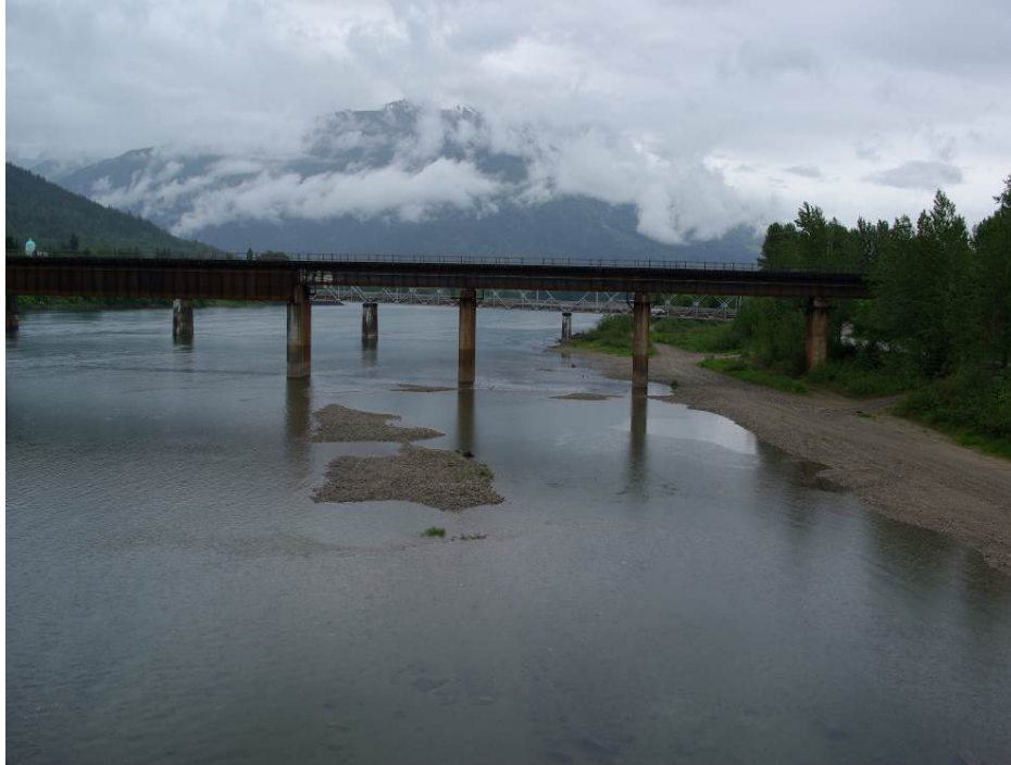
Photo 19. Overview of the Highway Bridge site on October 3, 2010 at approximately 1,000 m 3 /s discharge with no Arrow Lakes Reservoir inundation
