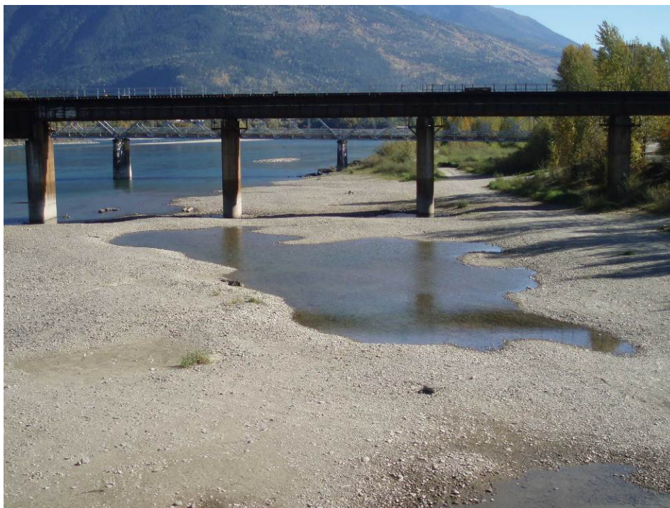
Photo 20. Overview of the Highway Bridge site on October 3, 2010 at approximately 400 m 3 /s discharge with no Arrow Lakes Reservoir inundation
