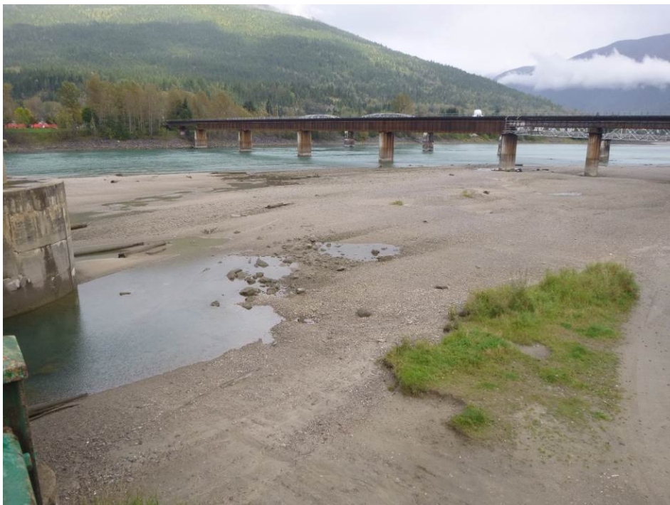
Photo 22. Overview of the Highway Bridge site on October 29, 2013 at approximately 200 m 3 /s discharge with no Arrow Lakes Reservoir inundation
