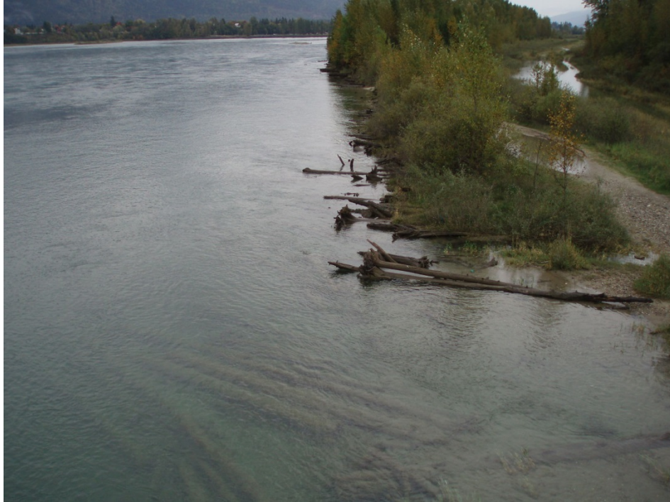
Photo 23. Overview of the Highway Bridge site at Area #3 on Oct 5, 2010 at approximately 400 m 3 /s discharge. The site is inundated by the Arrow Lakes Reservoir.
