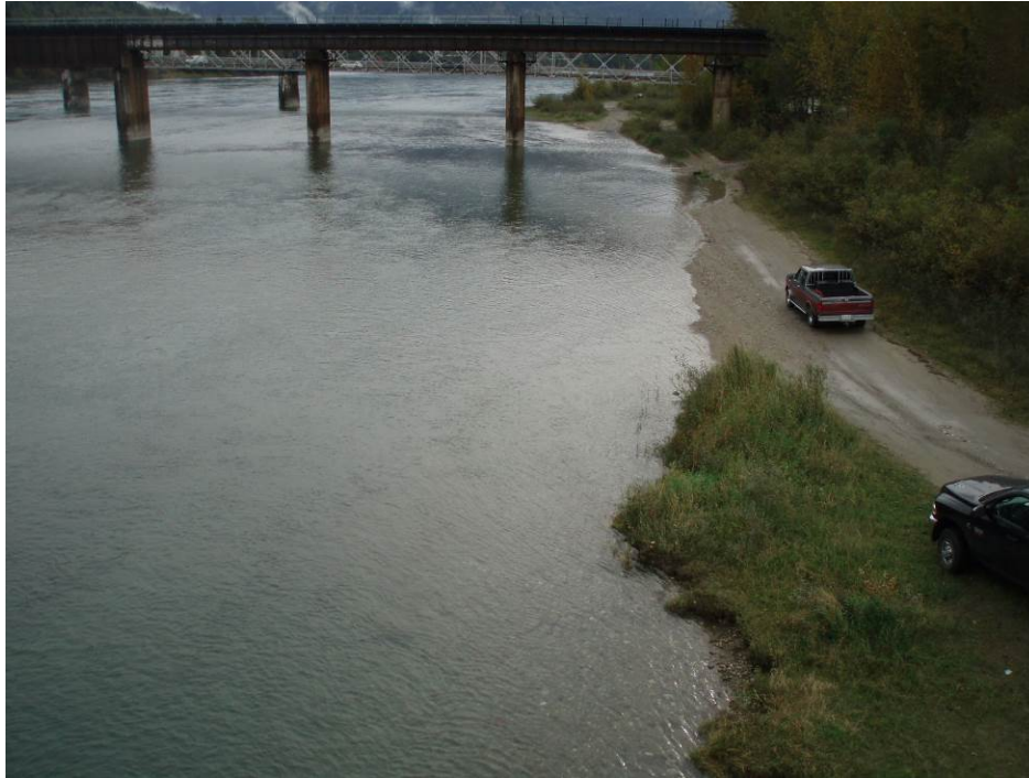
Photo 17. Overview of Highway Bridge site at Area #1 on October 6, 2011 at a discharge of approximately 800 m 3 /s. The site is inundated by the Arrow Lakes Reservoir.
