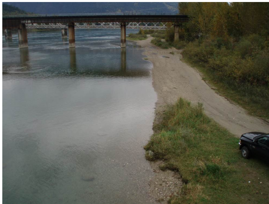
Photo 18. Overview of Highway Bridge site at Area #1 on October 6, 2011 at a low discharge of approximately 200 m 3 /s. The site is inundated by the Arrow Lakes Reservoir.
