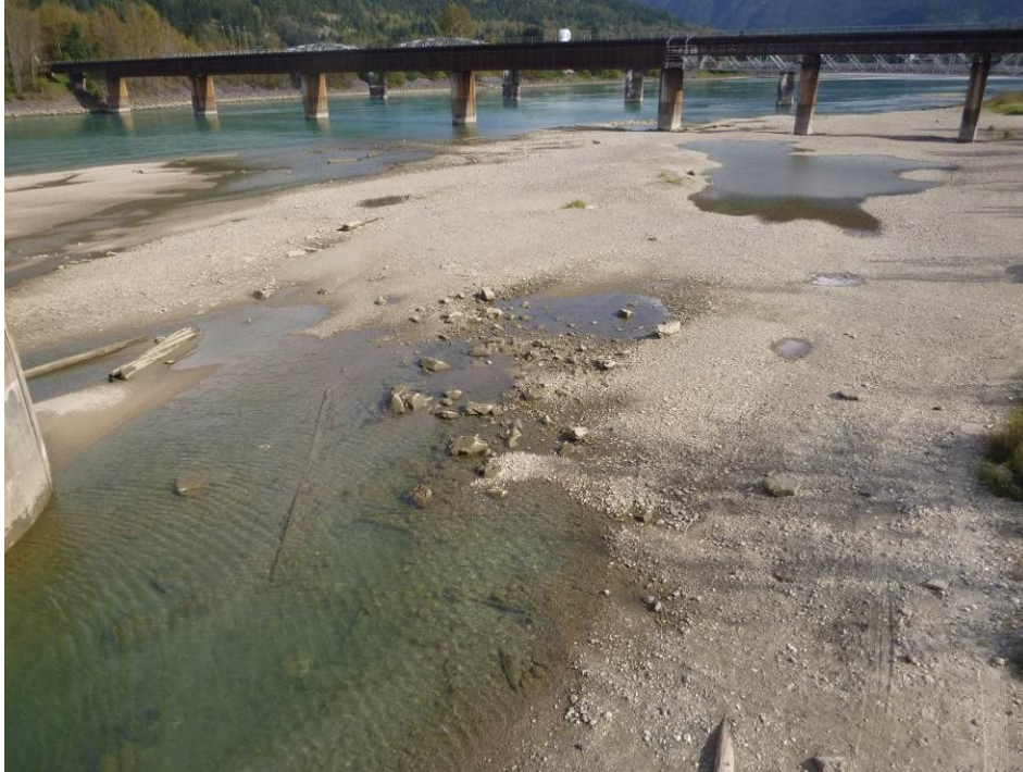
Photo 21. Overview of the Highway Bridge site on October 29, 2013 at approximately 400 m 3 /s discharge with no Arrow Lakes Reservoir inundation
