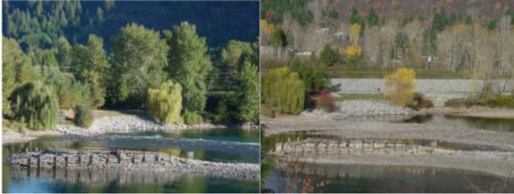
Figure 6-1: The view looking from the south bank of the Columbia River towards the Castlegar waste water treatment plant prior to (left panel) and during (right panel) construction. Construction activity in the fall of 2014 removed extensive vegetation along the sewage lagoon berm as well as reinforcing the berm with rip-rap (visible in right panel). Note the proximity of Breakwater Island in the foreground to the construction area behind. Such activity may have affected the distribution of herons in the Waldie Island area during the winter of 2014/15. Photos © Walter Volovsek
