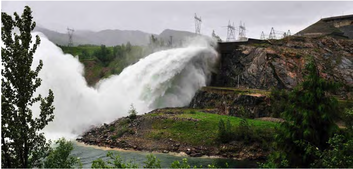
Figure 4-3: The Revelstoke Dam spilling (June 17, 2012)
