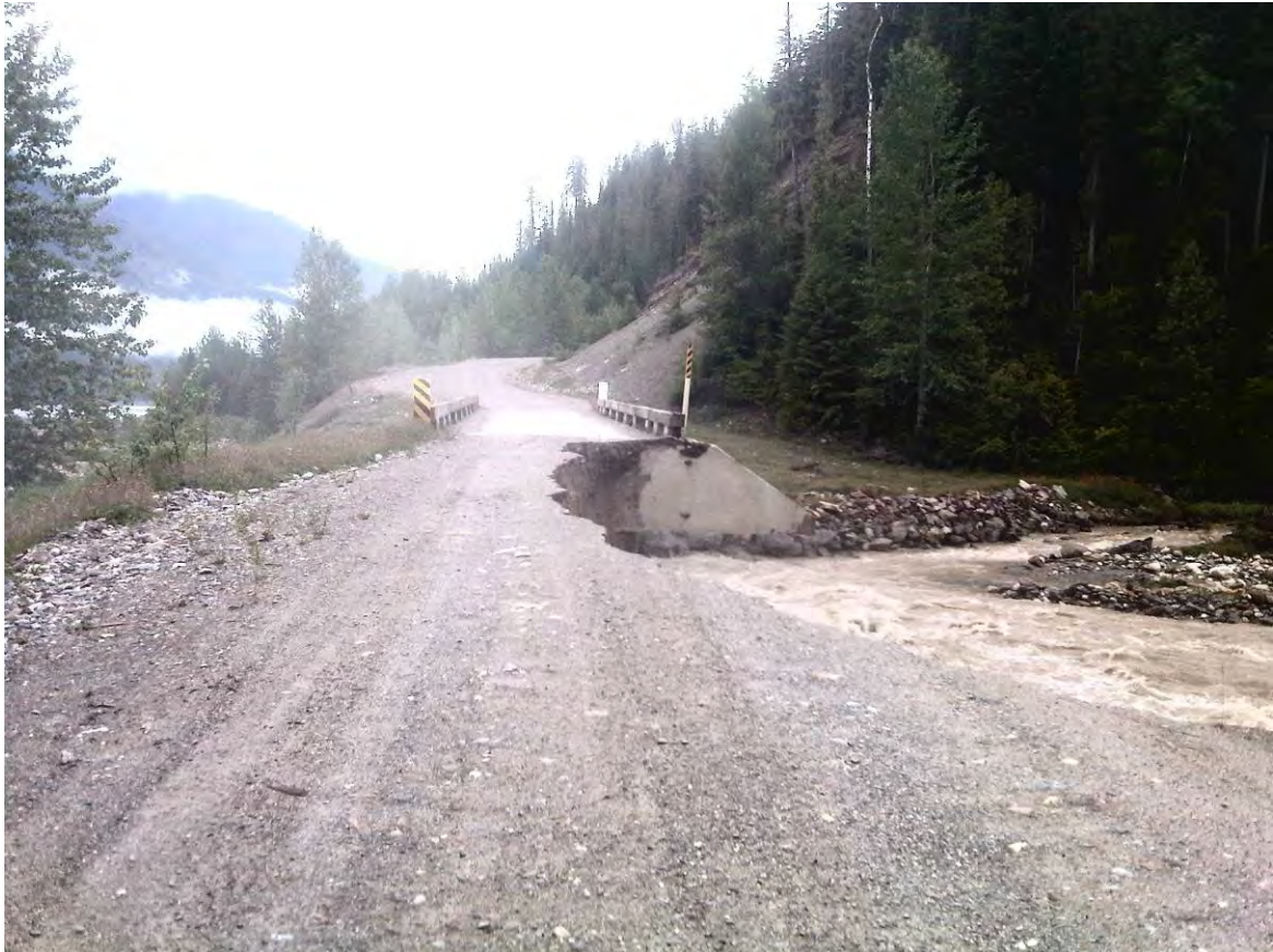
Figure 3-4: Example of a road washout in June (Prattle/Chatter Creek area), photographed as the road was eroding. This extended rain event caused many washouts in B.C. and a premature ending to nest monitoring in that study area in Bush Arm in 2012 (photo Jen Greenwood).
