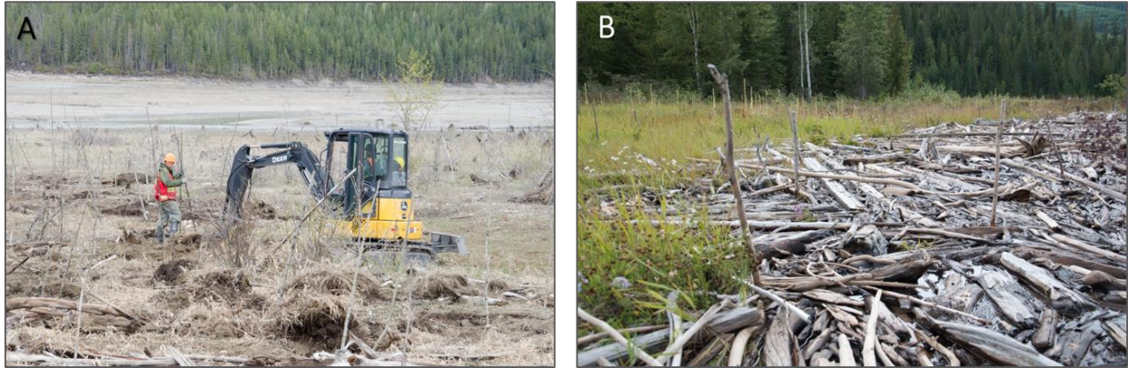
Figure 4-9. Examples of revegetation prescriptions trialed at Goodfellow Creek in 2008. A: shrub stakes (machine planted) and B: shrub stakes surrounded by wood debris in 2011. Photo credit: Doug Adama.
