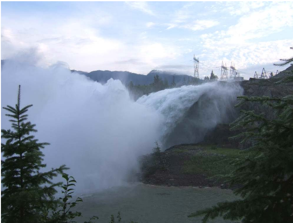
Spilling 40kcs at Revelstoke Dam, July 15, 2012
