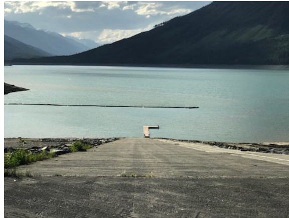
Figure 14. Bush Harbour high water after
