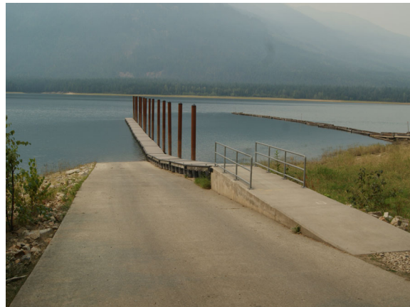
Figure 20. Burton South after
