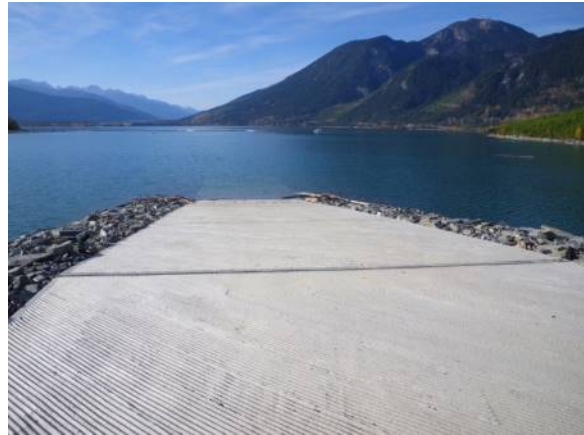
Figure 14. Bush Harbour high water after
