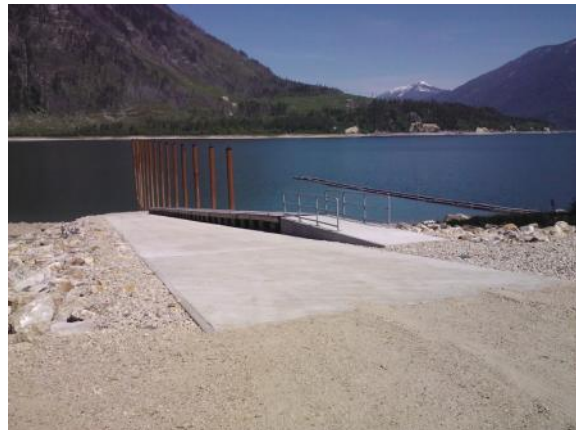
Figure 20. Burton South after
