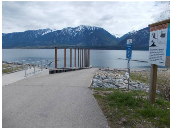
Figure 30. Shelter Bay after
