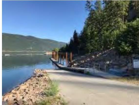
Figure 31. Anderson Point after
