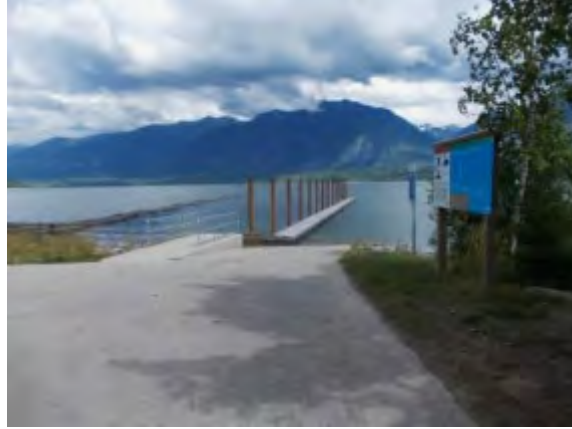
Figure 43. Shelter Bay after
