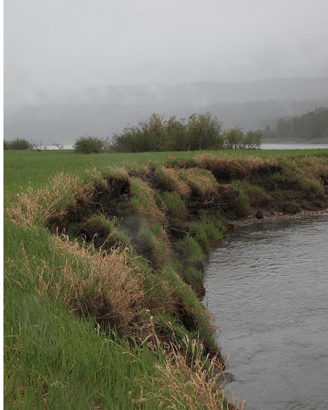
Figure 12. Sloughing of soils and vegetation near the Illecillewaet River (from Enns et al. 2012). In 2013, most of the clumps in the failure area had been washed away.
