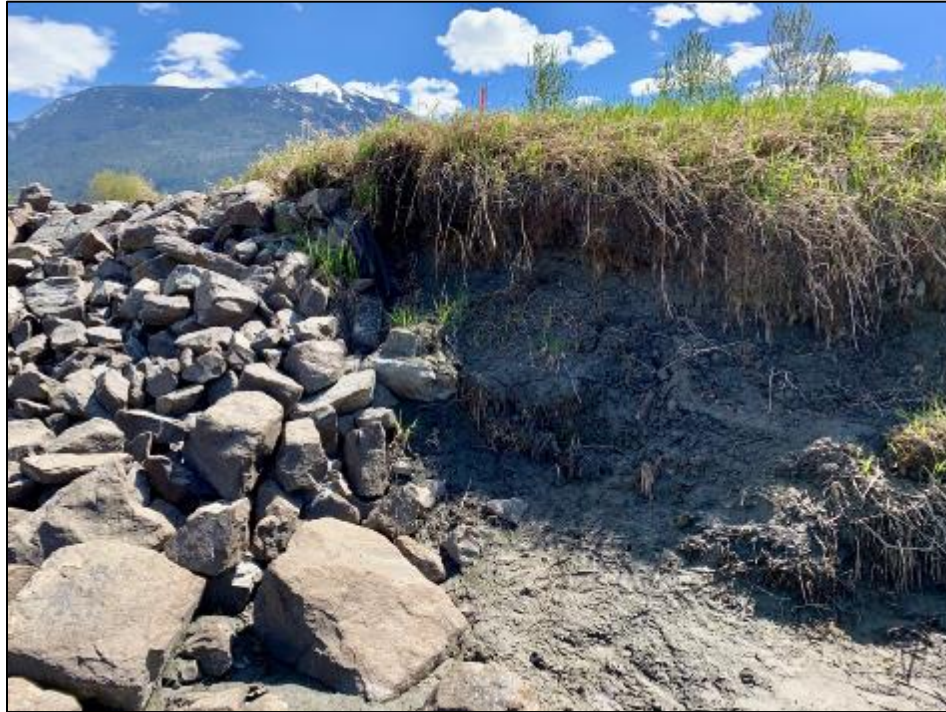
Figure 5-2: Undercutting of the bank at the mouth of the east channel of WPW-6A. May 9, 2019.
