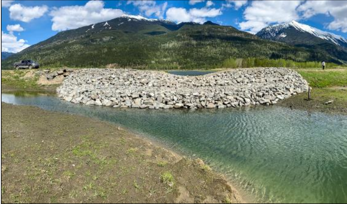
Figure 5-8: Image of the WPW-15A wildlife physical works at Cartier Bay. May 10, 2019.
