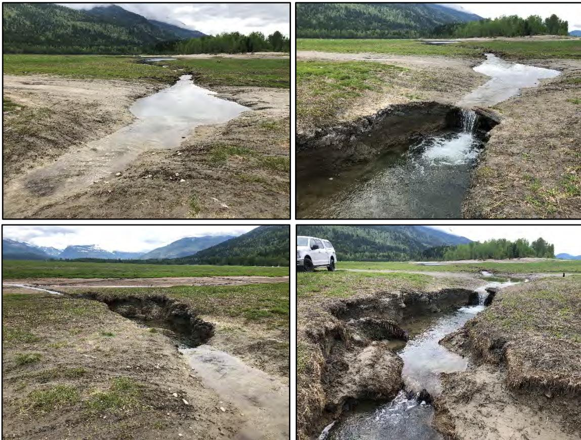
Figure 5-8. Overflow from the west compartment of Cartier Bay wetland where it crosses an access road near WPW-15A, with associated erosion channel and head-cut adjacent to the road. Photographed 15 May 2020.
