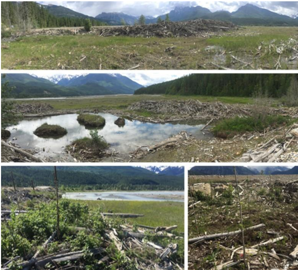
Figure 6-25: The Bush Causeway North treatment site showing mounds, cleared ponds, establishing vegetation on mounds (bottom left), and live stakes (bottom right). Photos were taken June 18, 2017.
