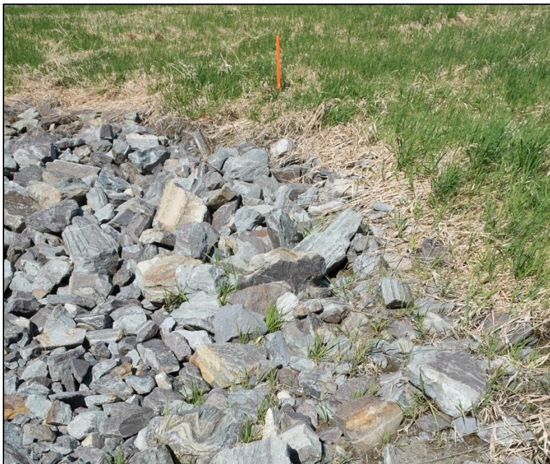
Photo 1601B. Integration of fines and vegetation in the riprap.
