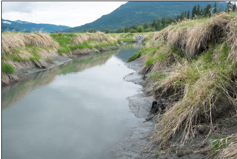
Photo 1601F. Slumping in the main channel.
