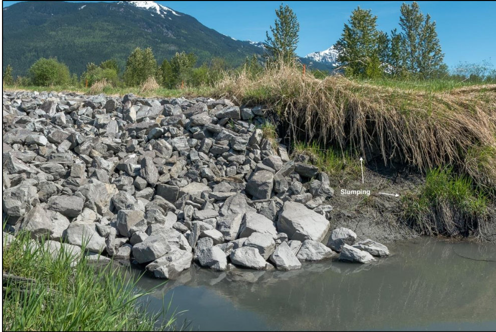
Photo 1601C. Slumping at the southwest corner of the channel.
