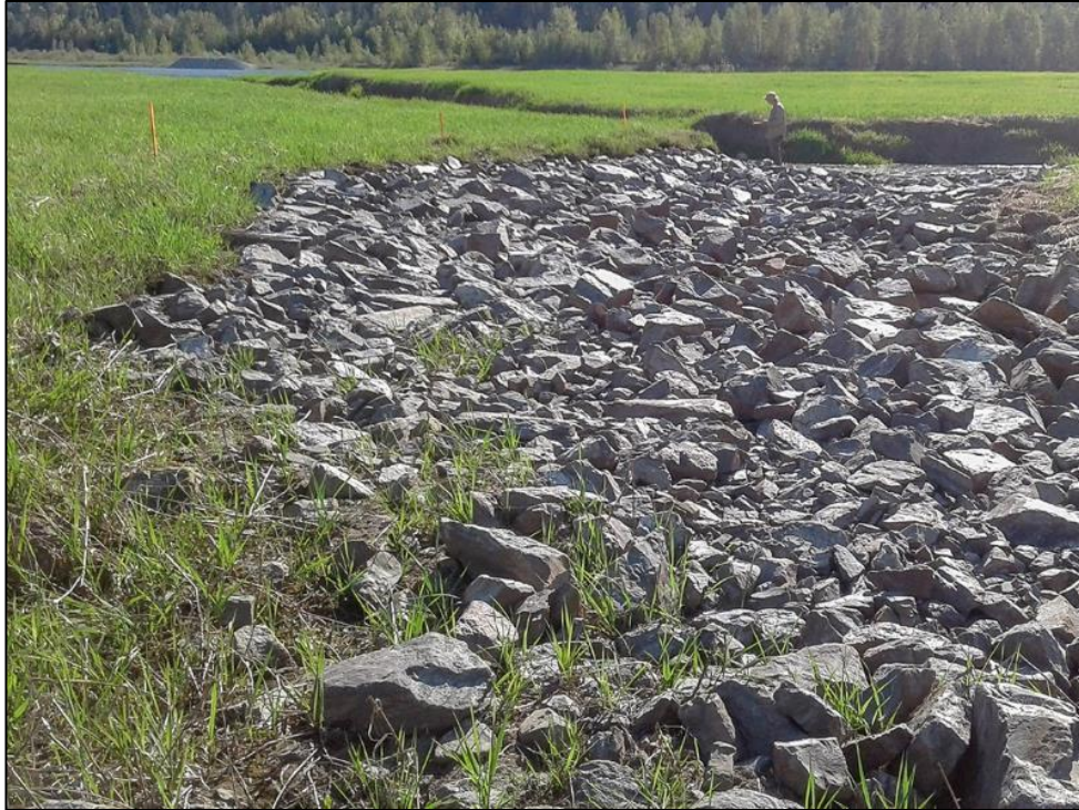
Figure 5-1: Reed canarygrass (in the foreground) ingressing into the riprap along the margin of the WPW-6A east erosion channel, May 2018.
