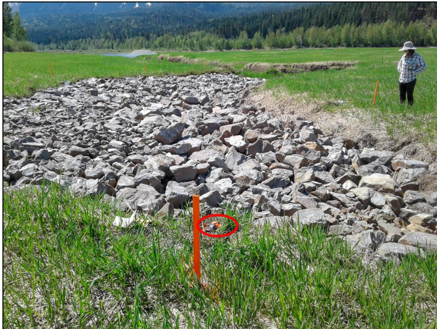
Figure 4-1: East erosion channel at WPW-6A, May 2018 The stake in the foreground is 122 cm behind pin 1-5 located at the margin of the riprap – channel bank interface (circle).
