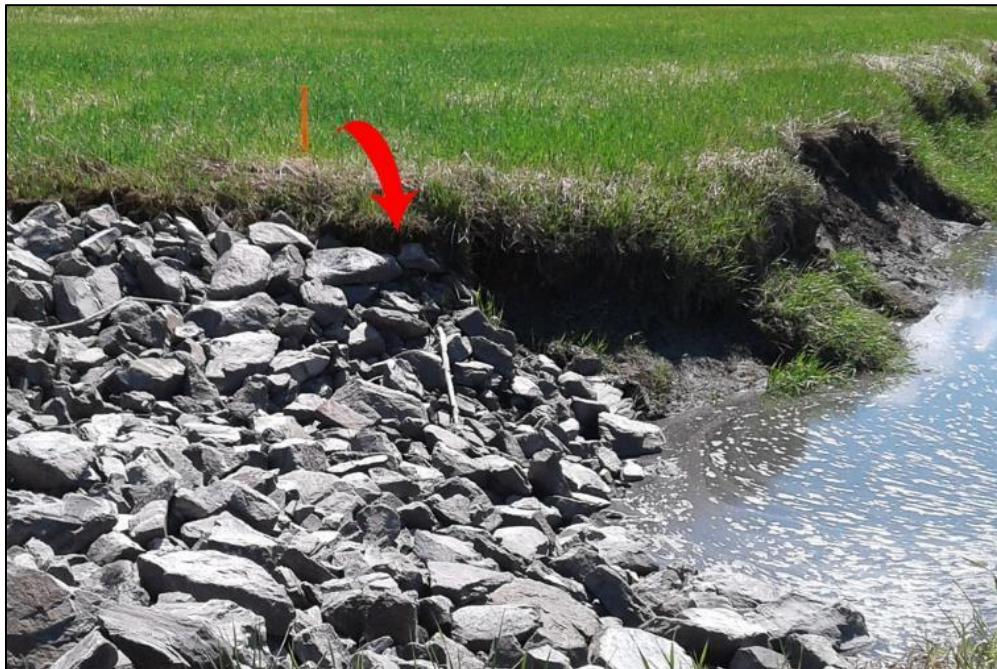
Figure 5-2: Soil movement, slumping, and bank undercutting at the mouth of the east channel of WPW-6A, May 2018. The arrow indicates the location and direction of soil movement and slumping.
