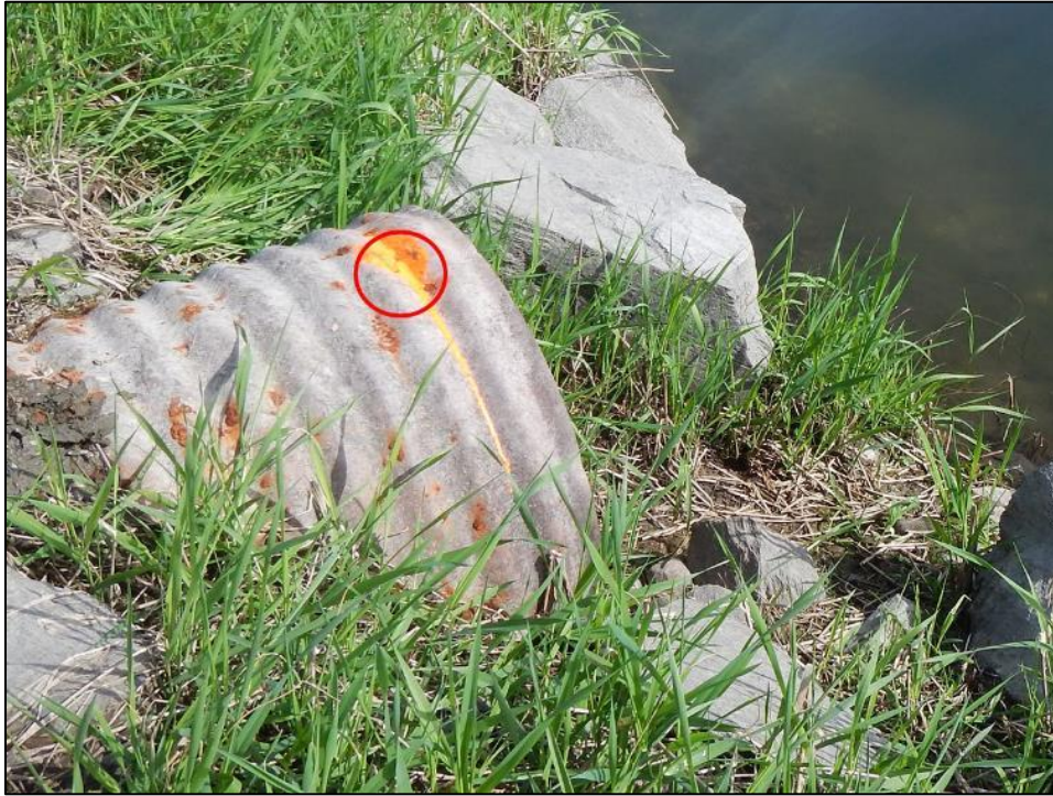
Figure 4-3: Location of survey reference point CS15A established by Waston Engineering on a culvert near Site 15A.
