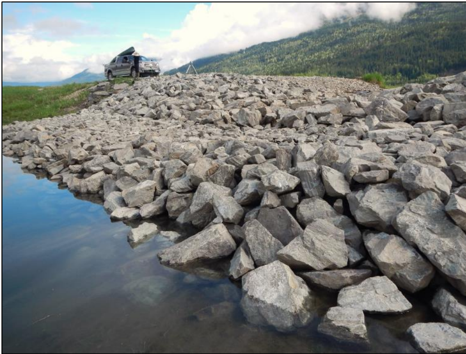
Figure 5-7: Images of the WPW-15A wildlife physical works at Cartier Bay, May 2018.
