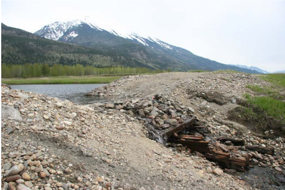
Photo of the collapsed box culvert in abandoned railbed that creates Cartier Bay wetland.
