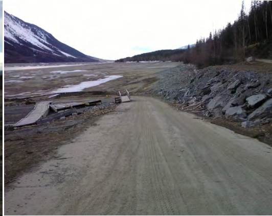
Figure 10. Construction at Valemount 2011
