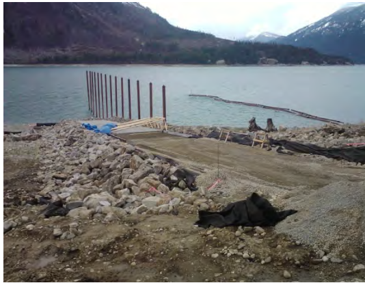
Figure 3. Burton South under construction.
