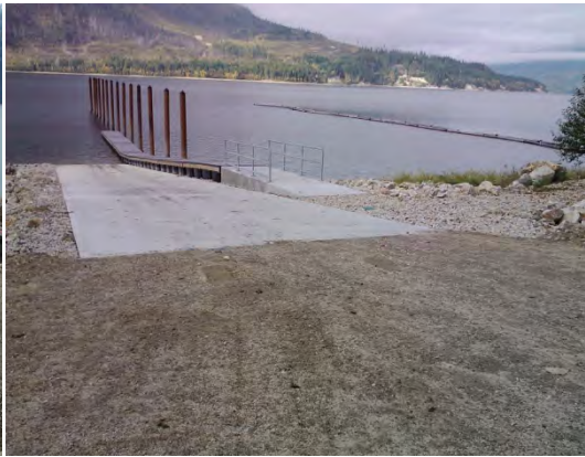
Figure 4. Burton South substantially completed with traffic counter installed.
