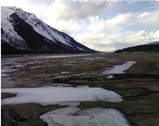
Figure 9. Prepping the ground for construction, Valemount Boat Launch
