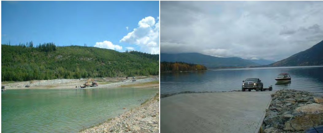
Figure 1. Before and after photos showing new boat ramp construction at Bush Harbour.
