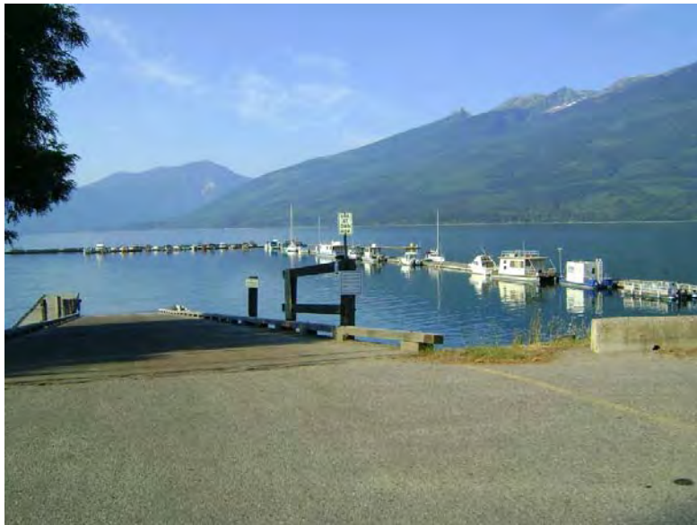
Figure 16. Nakusp boat ramp was the busiest of the sites, with 48% of traffic in 2010.
