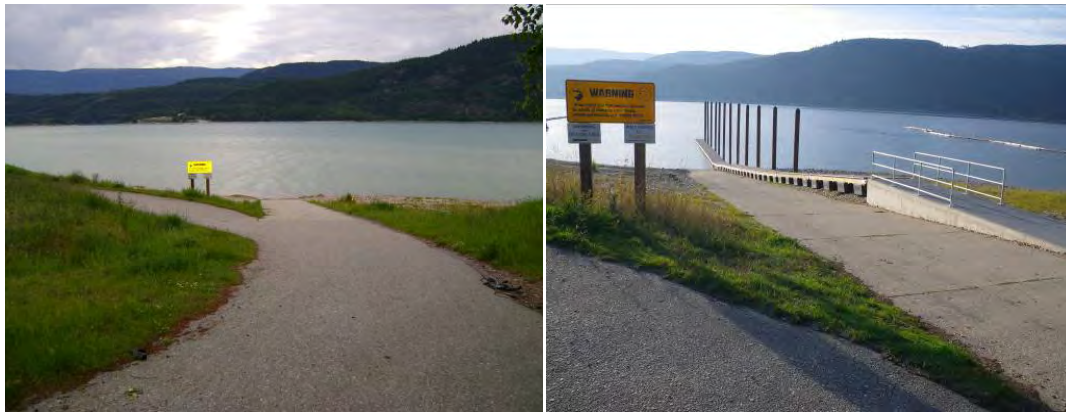
Figure 20. Before and after photos showing improvements at Fauquier boat launch.
