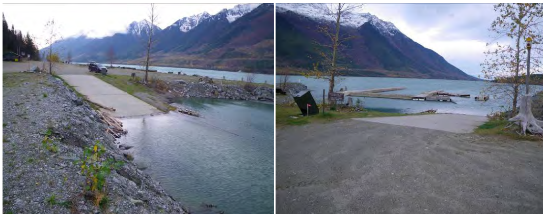
Figure 2. Boat ramp at Valemount, October, 2010.
