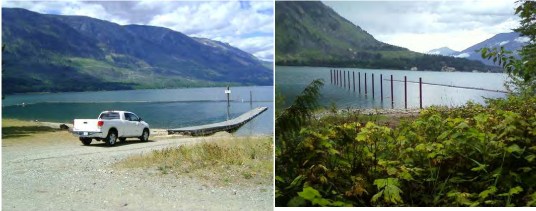
Figure 22. Photos showing Burton Historic Park boat launch, and new construction south of town.
