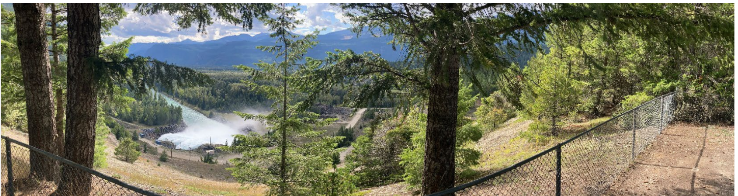
Duncan Dam from the lower viewpoint
